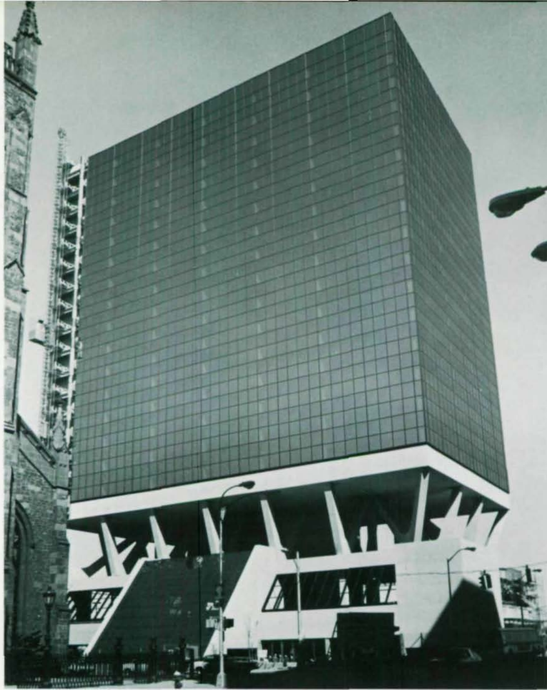
Dramatic One Corporate Center building, Hartford, Conn. "lands" on municipal garage on steel legs.
