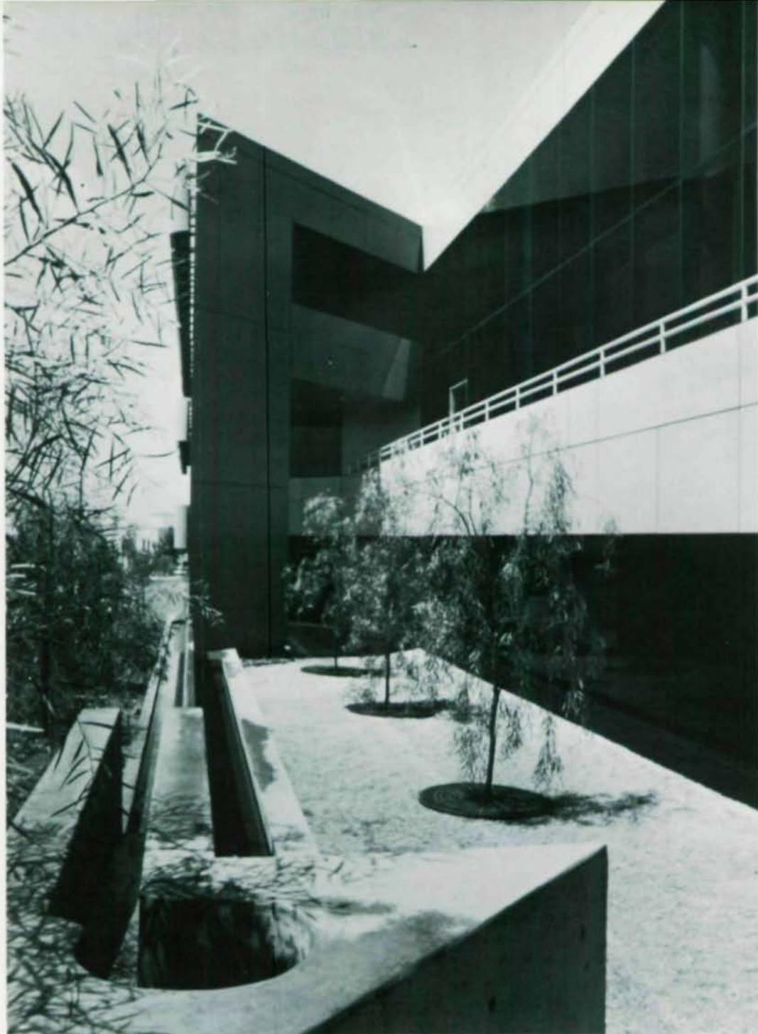
Southwest Forest Industries' new corporate headquarters in Phoenix, Ariz. boasts panoramas in all directions. Building was sited to take full advantage of environment.
