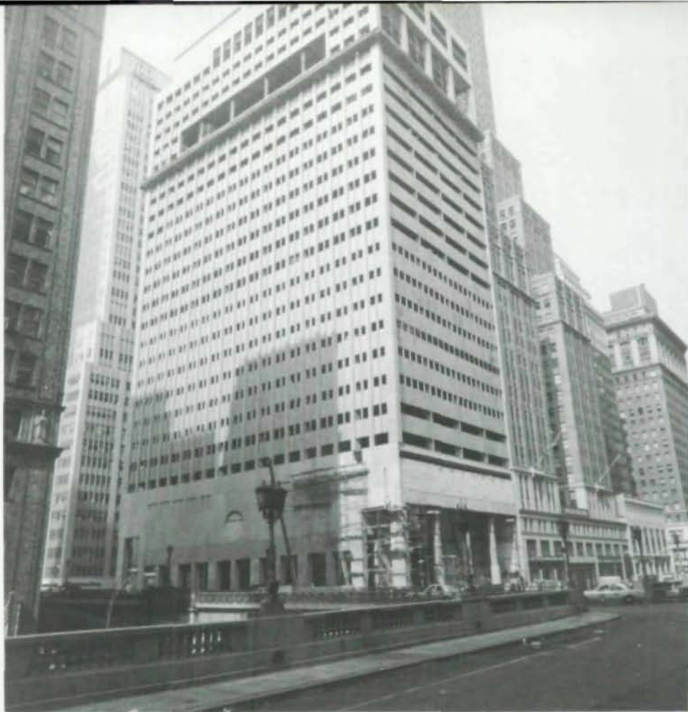
New Philip Morris Building in busy Manhattan. Far below (bott. photo) two subway systems rush within inches of steel girders erected, creating unique problems in fabrication and erection.
