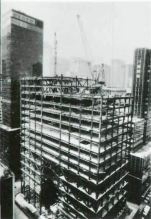
Early progress photos of steel framing of 112-ft high arch that fronts on Madison Avenue.
