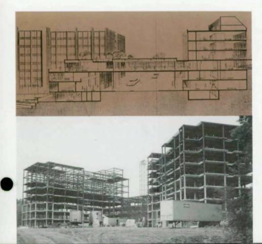
Steel framework was architect's choice for fast erection, flexibility of framing, reduced construction and financing costs.
