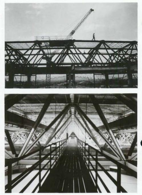
Truss system provides ample room for large duct system to feed through it, reduces building cubage and gives maximum head room for athletic events.
