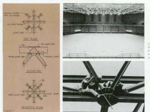
Unique roof framing system of 264 x 288-ft fieldhouse employs two-way pyramidal truss and special design hub connections.
