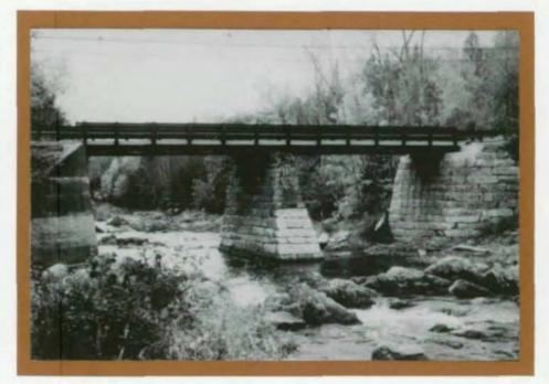
Rural one-lane bridge in Cornville, Me. Complete superstructure, with new weathering steel and rail system, was built for \$51,000.
