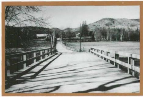
Before—one-lane bridge at Carthage, Me. prior to reconstruction (top); After—bridge was reconstructed with reclaimed steel beams and timber floor for \$33,000.
