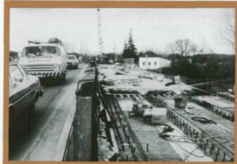
Deteriorated deck (top) was reconstructed (bott.) using half of bridge width to maintain traffic.
