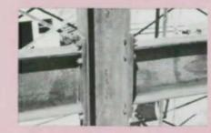
Closeups detail K-bracing (L) and spandr end plate design (below) Photos courtesy LLLs Jeune Co
