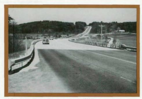
U.S. Route I bridge. Woolwich Me was originally built in 1934. New concrete deck was placed on existing steel and structure widened 19 It by extending existing substructure, adding new superstructure.
