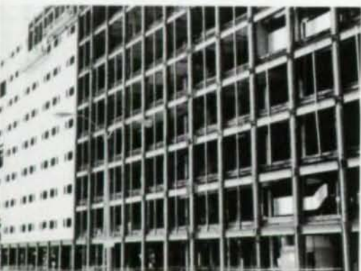
Sequence of construction: (l. above) near end, new exterior moment frame; mid-section, existing steel frame after masonry wall removal; far end, new cladding over new steel frame. Note sequence (l.) of cladding installation is left to right, not bottom up.
