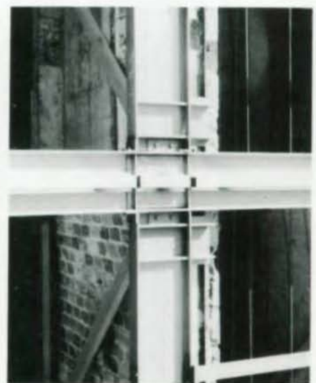
Existing riveted built-up column spandrel detail (l. above); above, new all-welded column/spandrel.
