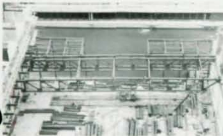
Figure 3—"The Box" under construction
