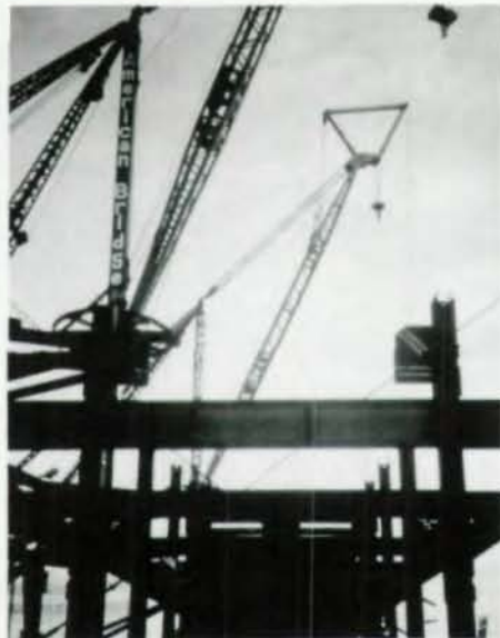
Steel erectors at upper core level
