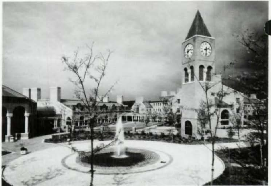
Beneficial Center, Peapack-Gladstone, N.J.—firm's largest project to date.
