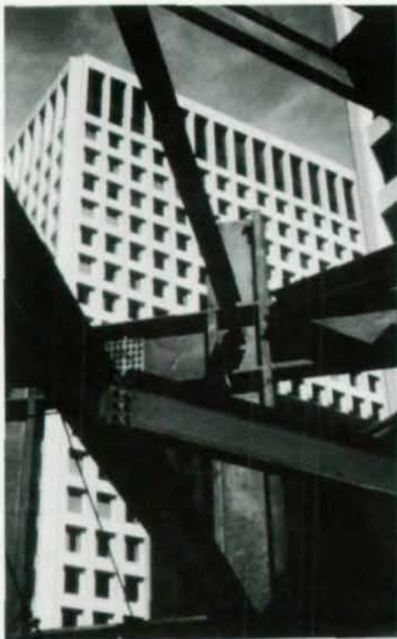
Interior floor framing/tree column, with Two Allen Center in background
