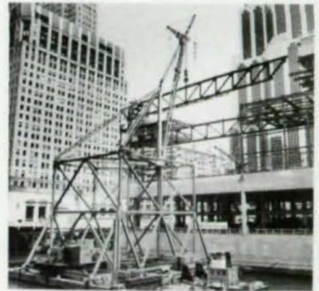
Water-borne crane lifts 175-ft, 65-ton truss into position.
