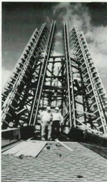
Central skylight and cupola (above and top r.) employ tension and compression rings at bottom and top chords of trusses.
