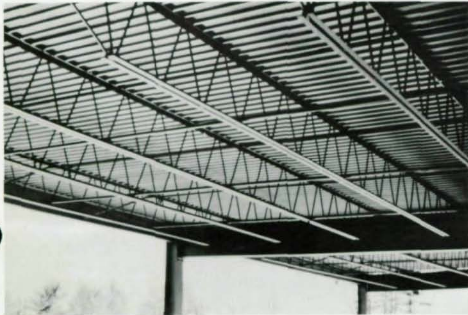
Typical construction of roof deck, steel joists on steel framing
