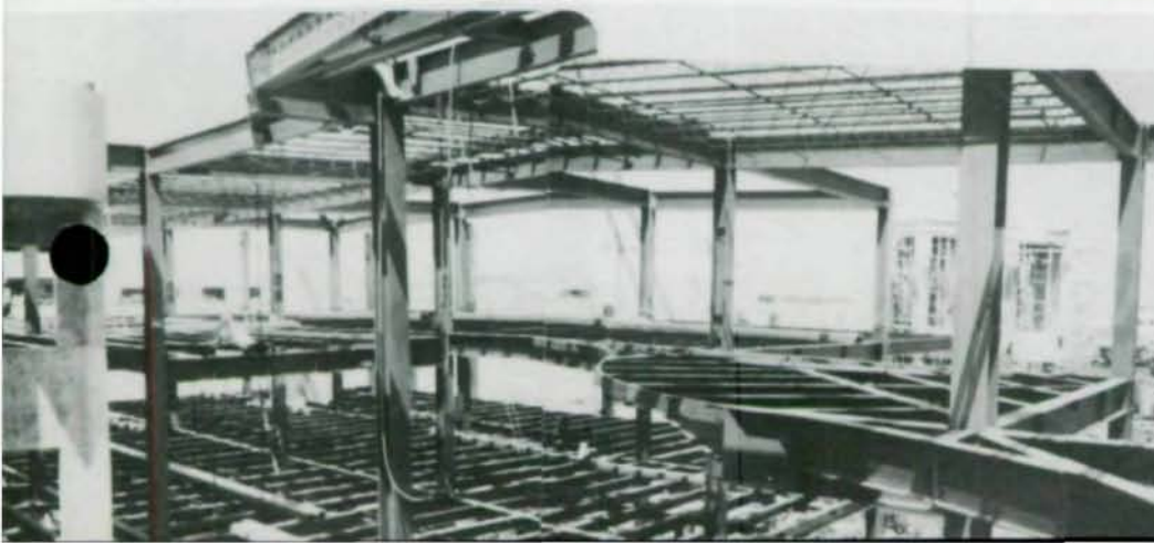
Composite photos show framing around open atrium (above) and future glass-enclosed elevator areas.
