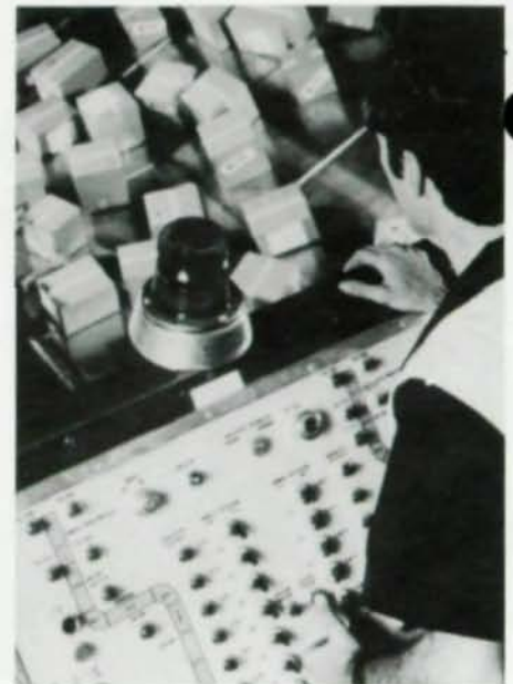
Computer-assisted conveyor system sorts over 1.5 million pounds of cargo nightly.
