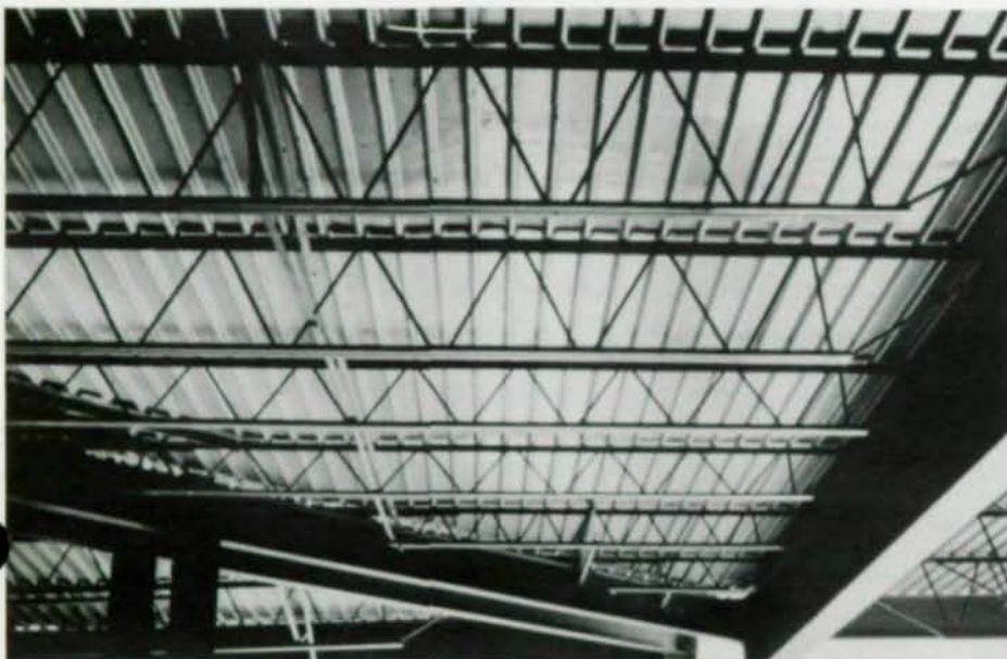
Roof deck, joists and framing
