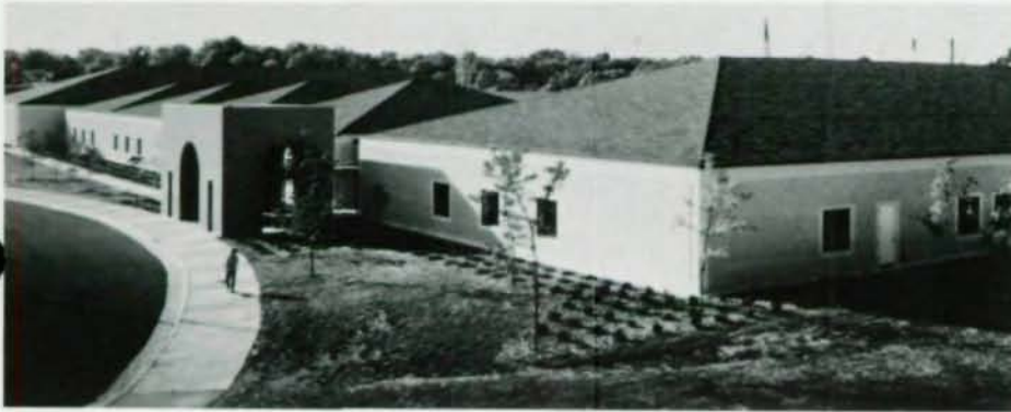
Kannapolis (N.C.) Middle School arranges eight academic modules around landscaped courtyards. Distinctive roof lends human scale to one-story structure. Steel beams and bar joists form roof of rectangular modules.
