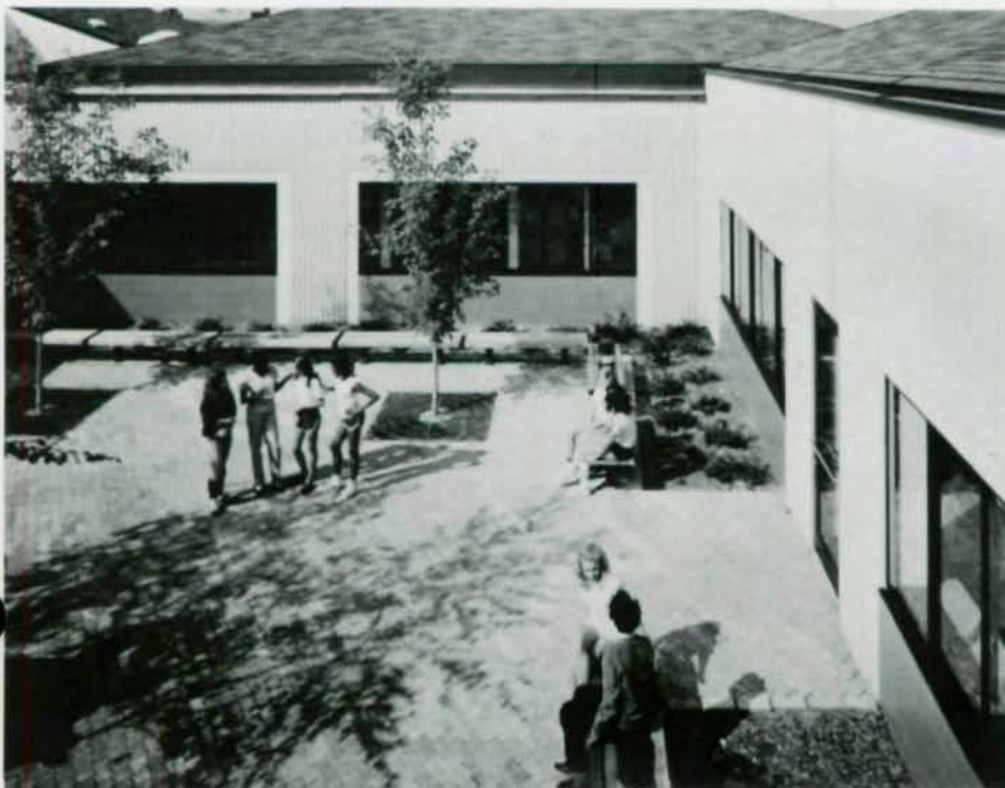
Kannapolis (N.C.) Middle School arranges eight academic modules around landscaped courtyards. Distinctive roof lends human scale to one-story structure. Steel beams and bar joists form roof of rectangular modules.
