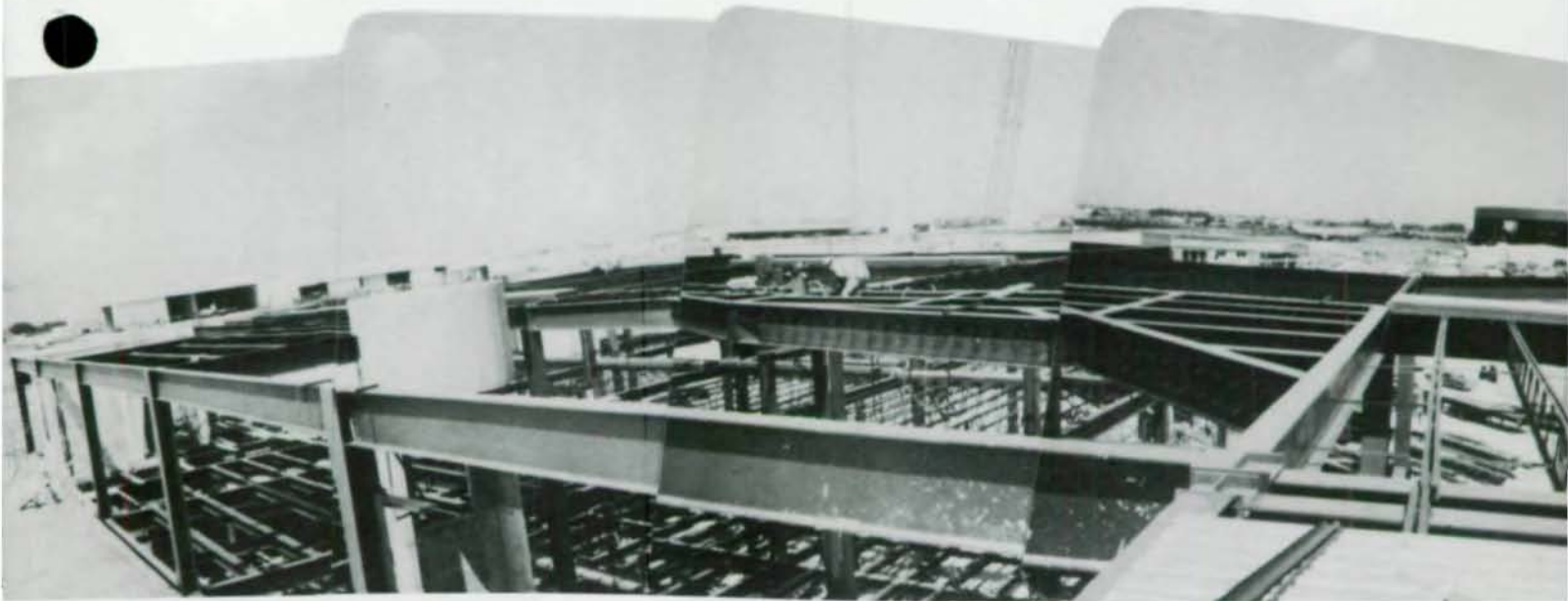
Composite photos show framing around open atrium (above) and future glass-enclosed elevator areas.
