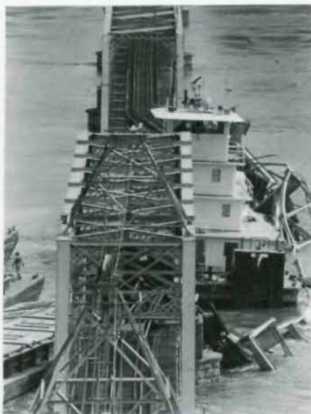
Runaway barges badly damaged Norfolk & Western RR bridge at Hannibal, MO.
