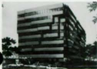
Greenspoint I, Houston, TX Arch: S.J. Morris Engr: Walter P. Moore & Co. Cont: McGregor Construction Co. Dvlpr: Friendswood Development Co. (Exxon)
