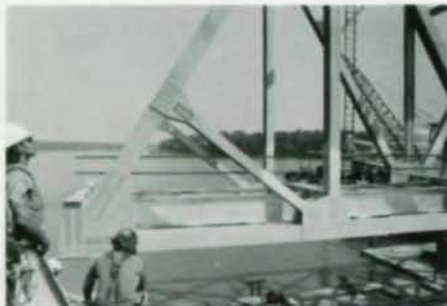
New truss is lifted to clear piers (above), swung into place and lowered onto bearings (l.). Total lift time: 45 minutes. Within six hours first train passed over new span.
