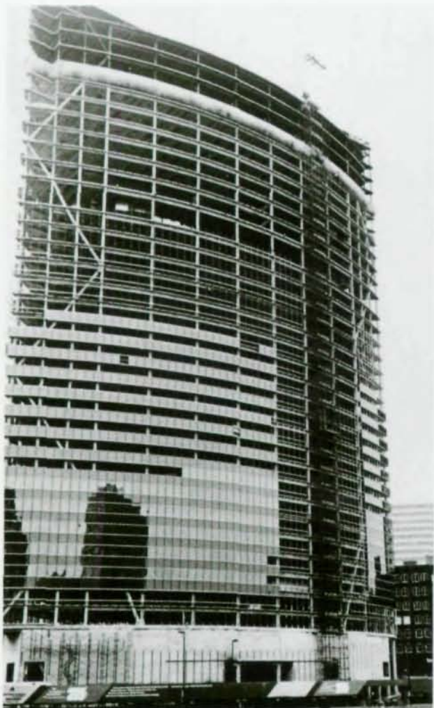
Last steel up for 333 Wacker Building at historic site (l.). Above (and r.) shows building's structural steel frame as it curves to adapt to triangular site. Renowned Merchandise Mart in background (r.).
