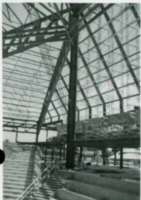
Photo 1 (above) is structural steel frame of roof. Long spans (up to 131 ft-6 in.) provide column-free areas for large auditorium. Photo 3 (above, l.) is exterior of steel frame, shows steep roof slopes at south and west faces.
