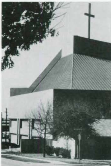
Exterior of Prestonwood Baptist Church, Dallas (l.) shows steel-framed roof sweeping upward to cross. Long truss spans in interior (r.) provide uninterrupted sightlines for worshippers.
