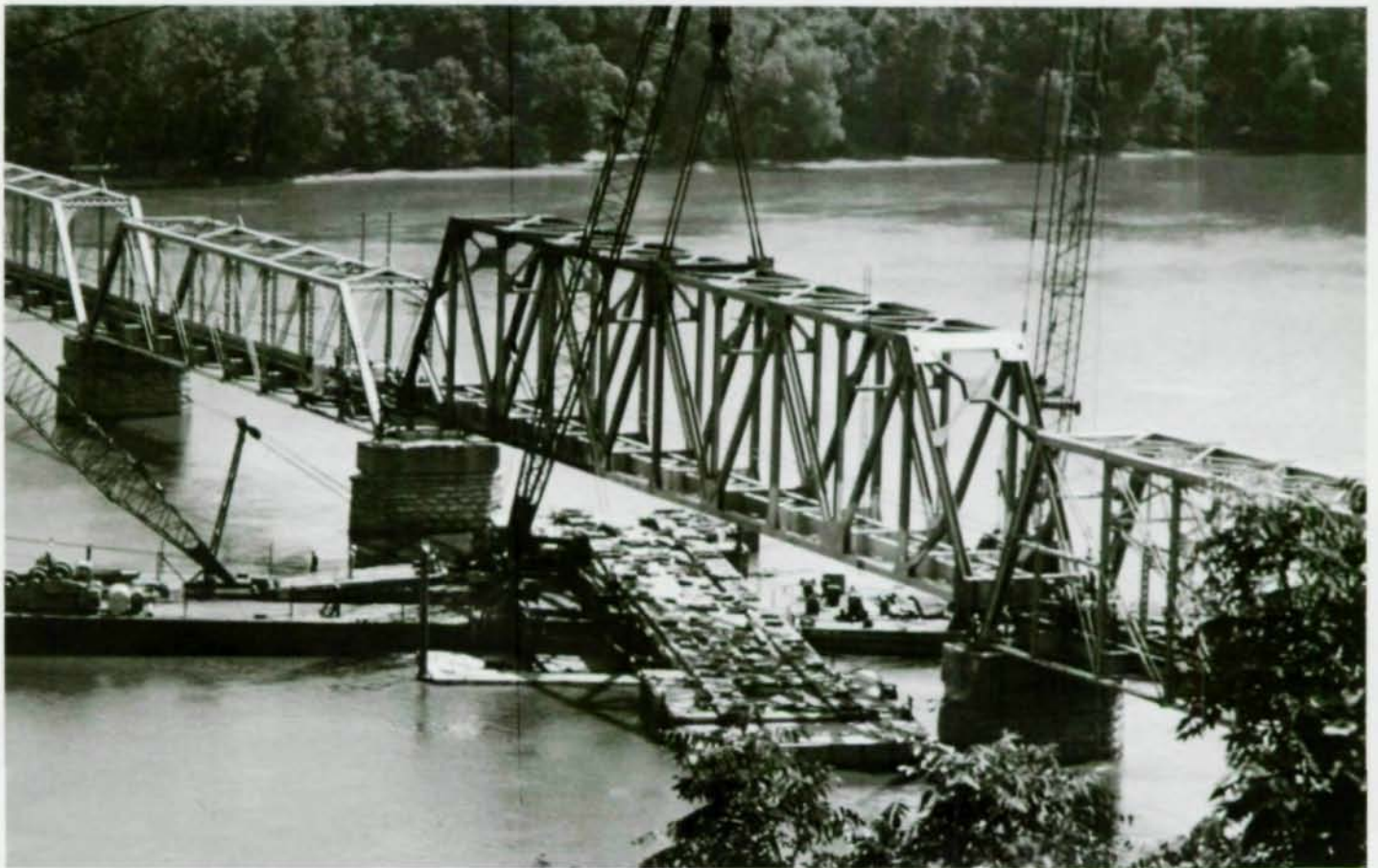
New truss is lifted to clear piers (above), swung into place and lowered onto bearings (l.). Total lift time: 45 minutes. Within six hours first train passed over new span.
