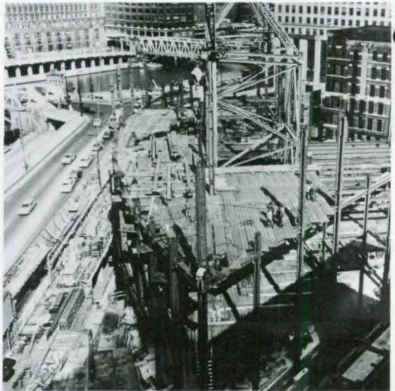
Last steel up for 333 Wacker Building at historic site (l.). Above (and r.) shows building's structural steel frame as it curves to adapt to triangular site. Renowned Merchandise Mart in background (r.).
