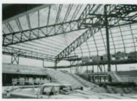
Photo 1 (above) is structural steel frame of roof. Long spans (up to 131 ft-6 in.) provide column-free areas for large auditorium. Photo 3 (above, l.) is exterior of steel frame, shows steep roof slopes at south and west faces.
