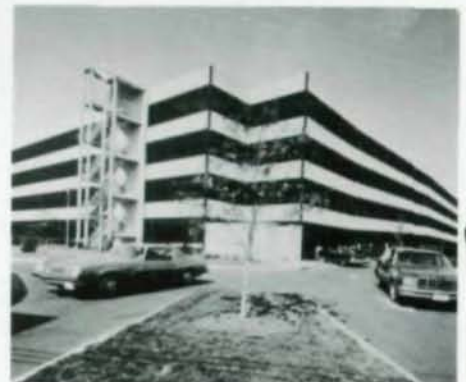
Parking deck for Roanoke Memorial Hospital (above, r.) sits on 30° slope. Cars enter at upper level, exit below.
