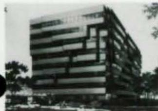
Greenspoint I, Houston, TX Arch: S.I. Morris Engr: Walter P. Moore & Co. Cont: McGregor Construction Co. Dvlpr: Friendswood Development Co. (Exxon)
