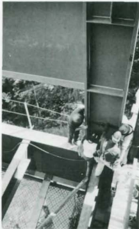
Workers fasten huge steel beams that link complex into one unit.
