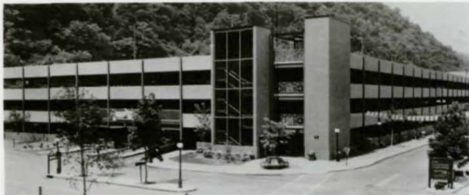
Located at popular Pittsburgh office, shopping, entertainment complex, 815-car Station Square garage uses exposed steel as prominent facade. Architect: Landmark Design.
