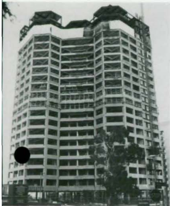
Mirabella Condominiums (L.) on posh Wilshire Boulevard's Golden Mile in Los Angeles. Distinct design, cost efficiency and seismic requirements dictated steel frame (below).
