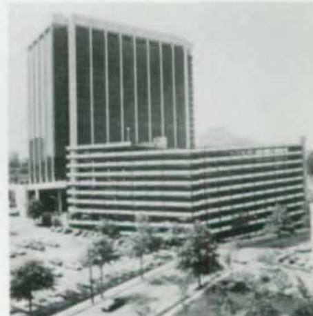
Eleven-story steel-framed parking structure in White Plains, N.Y. serves adjoining 23-story office building. Switching to steel saved $800,000. Architect: Seymour Gage.
