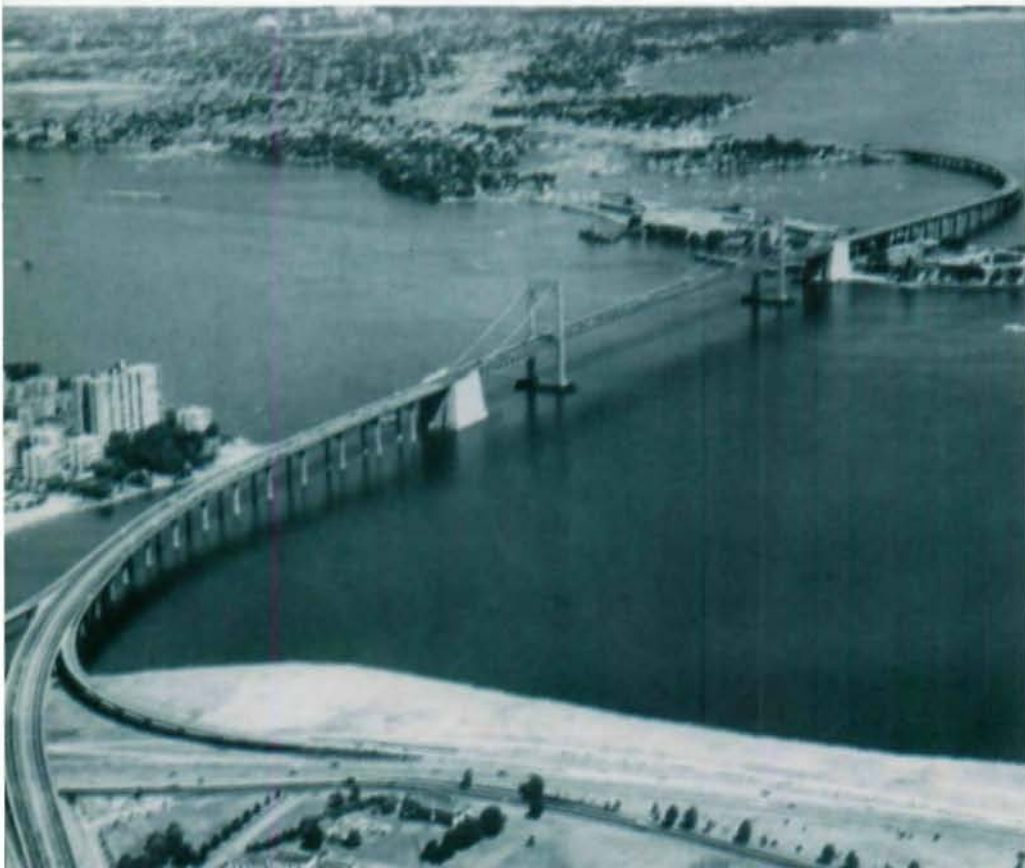
Throgs Neck Bridge, New York City, undergoes huge redecking program during 1984-85.
