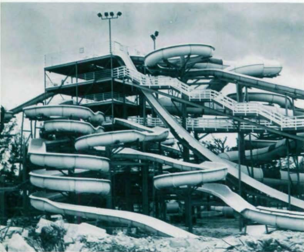
Figure 2. Unusual weaving and inter-looping of slides complicated design problems.
