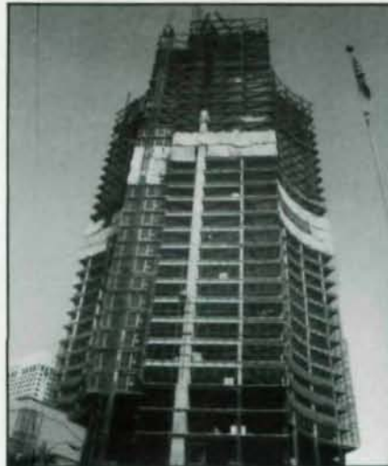
The new Columbia Center in Seattle, Washington will be 76 stories when completed, making it the tallest building west of Chicago. Owner & Developer: Martin Selig; Structural Engineer: Skilling, Ward, Rogers, Barkshire; General Contractor: Howard S. Wright & Company; Steel Fabricator: Samsung Corporation; Steel Erector: American Bridge, Division of U.S. Steel.
