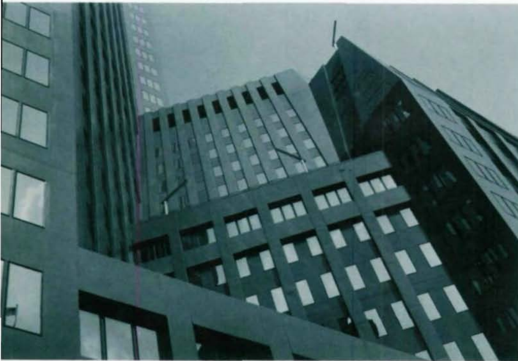
Top of "bustle" shows crisp details and numerous planes of stressed-skin facade.
