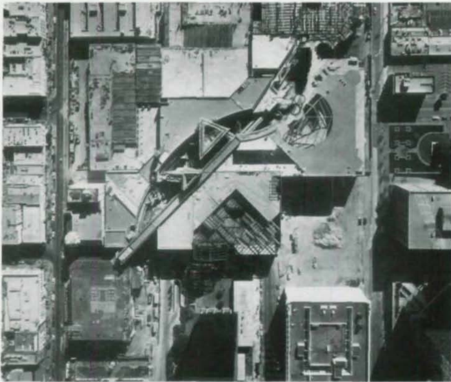
Model and aerial view reveal complexity of giant steel-framed structure.
