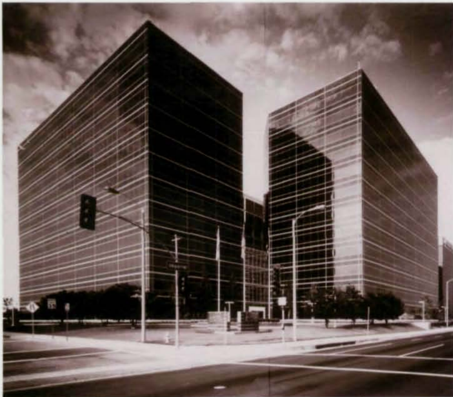
Twin 12-story Kilroy Airport Center towers, El Segundo, Cal. Exteriors were conceived as window walls uninterrupted by exposed structural steel members.
