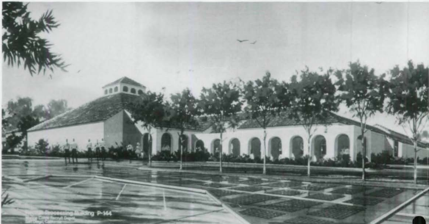
New Marine Corps Recruit Center, San Diego. Its large scale posed many engineering challenges.
