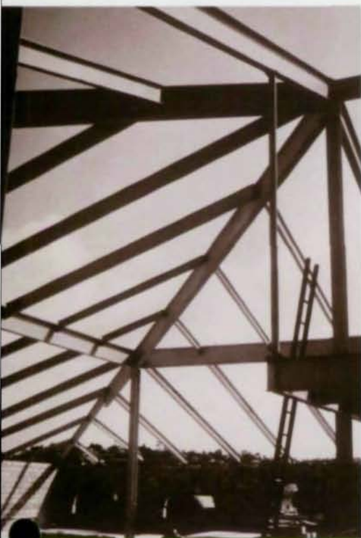
Steel-framed roof structure meets not only need for long spans but also desire for Spanish architecture.
