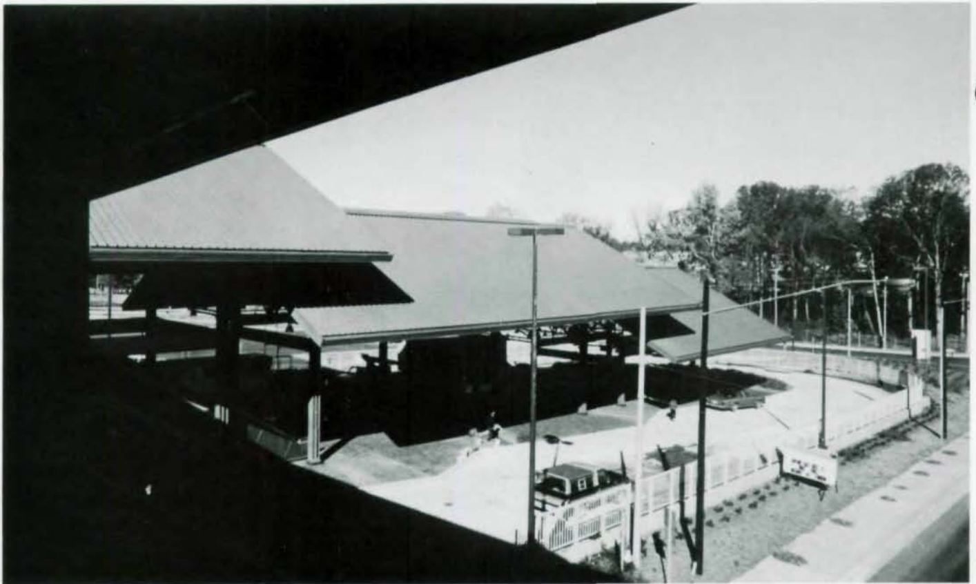
Station's suburban location called for gabled roofs similar to neighborhood housing. Gable permitted simple roof structure that was light and airy.
