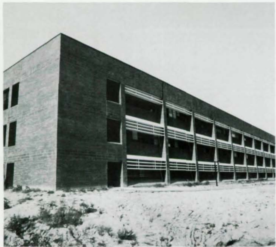
Customer Call Center was designed for maximum flexibility to meet future expansion needs. Steel framing permits movable walls, open planning and accessible service systems.
