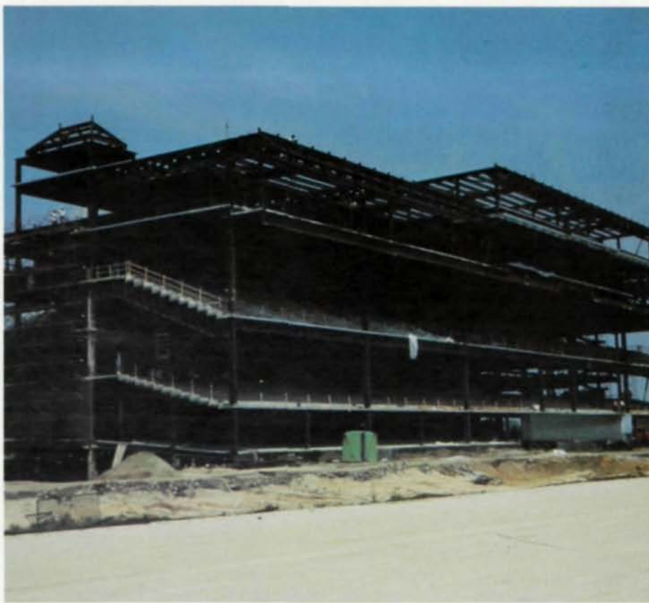
Grandstand/clubhouse structural frame at trackside
