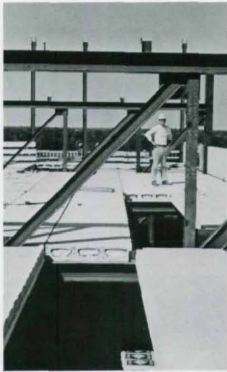
Close-ups of staggered-truss framing show diagonal and vertical members. Cost-saving, story-high trusses replace conventional beam-and-column framing and eliminate interior columns.
