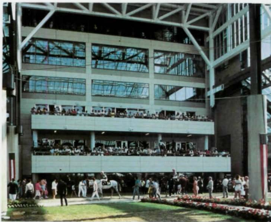
Crystal Paddock's glazed facade (above) supported by 27-in. valley beams. Below, clear-span space is created by exposed steel trusses of wide-flange shapes.
