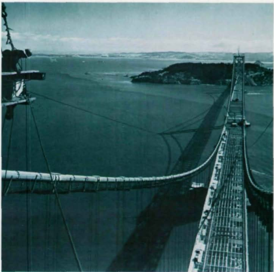
San Francisco-Oakland's famed Bay Bridge under construction, circa 1936.
