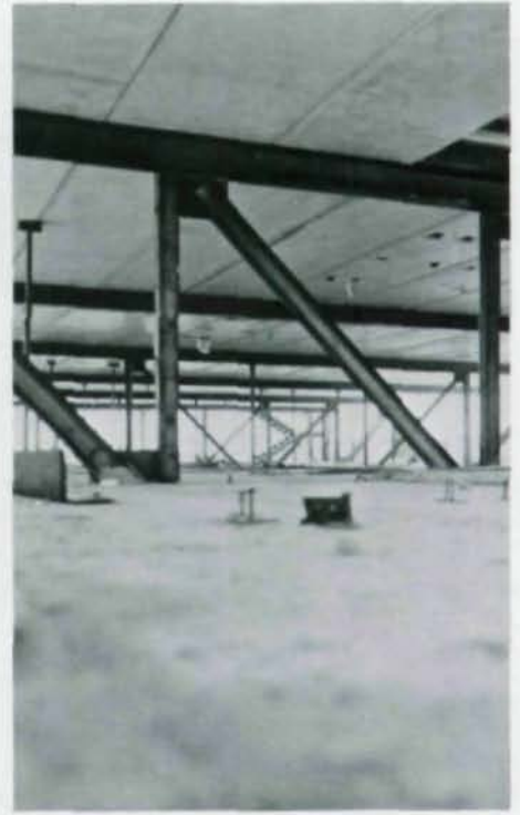
Close-ups of staggered-truss framing show diagonal and vertical members. Cost-saving, story-high trusses replace conventional beam-and-column framing and eliminate interior columns.
