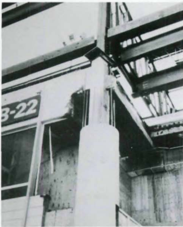
Old concrete column (l.) was strengthened by pouring concrete and compositing with existing to form new column. Detail of column strengthened by new steel jacket (above).
