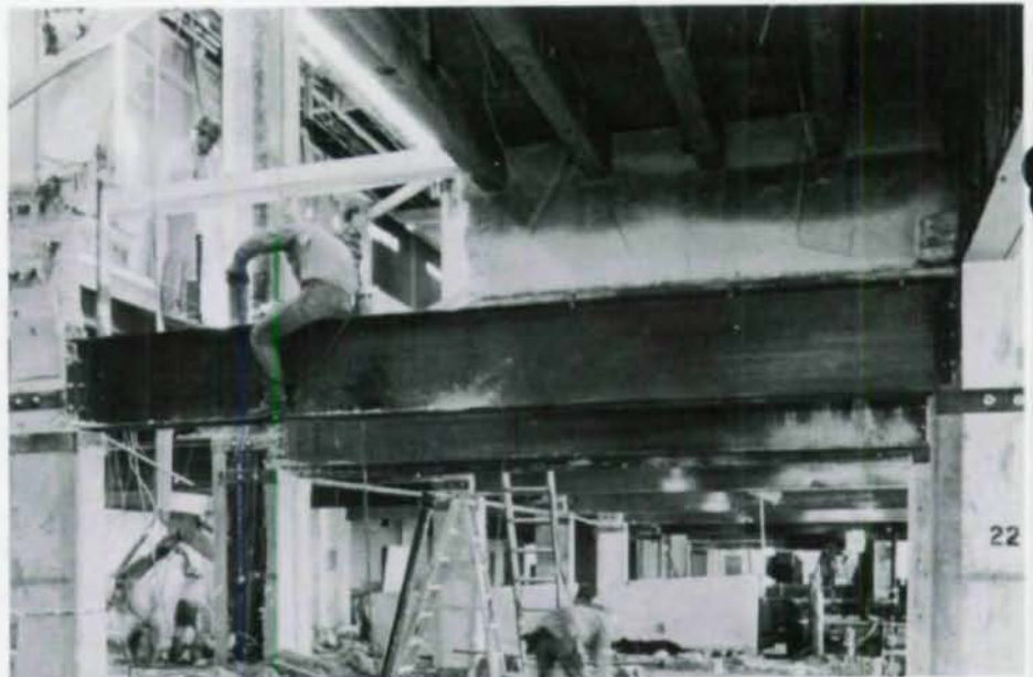
New permanent steel beam supports existing concrete beam and floor to accommodate moving walkway.
