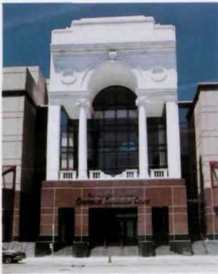
Reconstruction of arched marble facade of RKO Albee Theatre demanded exacting construction techniques.
