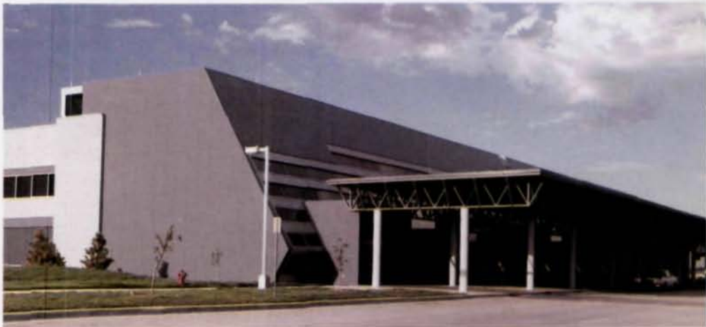
Exposed structural framing on separate front canopy is steel roof deck over standard joists, supported by custom-designed trusses.
