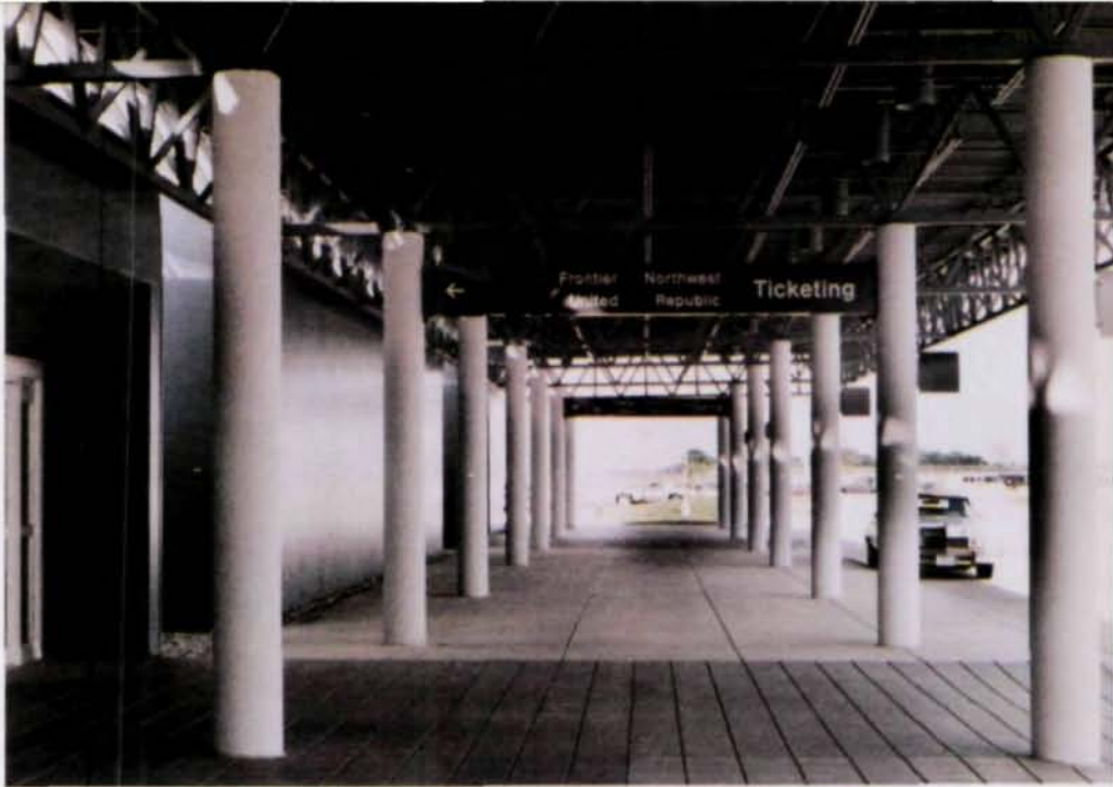
Exposed structural framing on separate front canopy is steel roof deck over standard joists, supported by custom-designed trusses.
