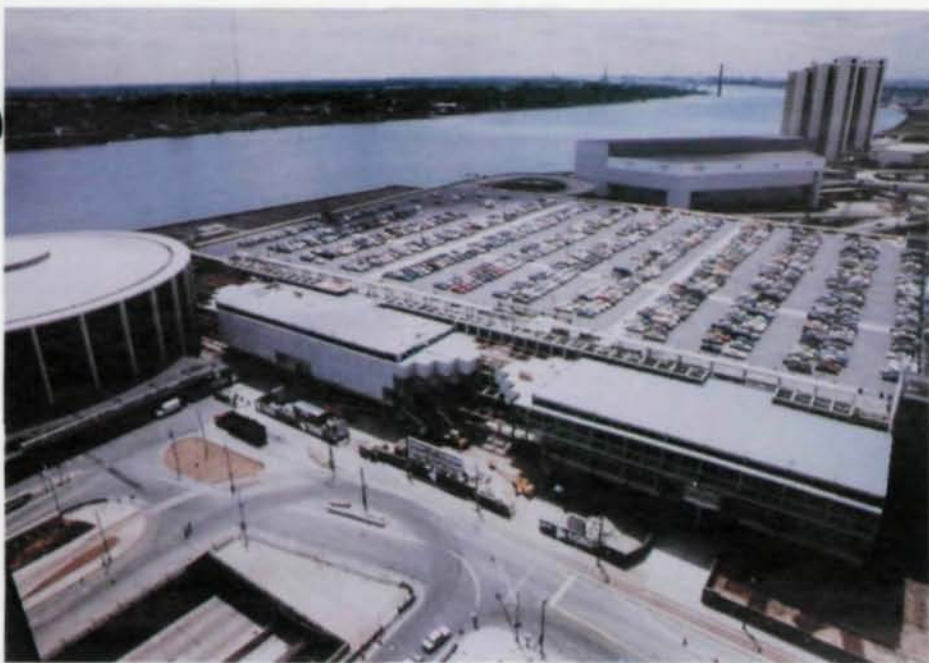
East side expansion, existing Cobo Hall, rooftop parking
