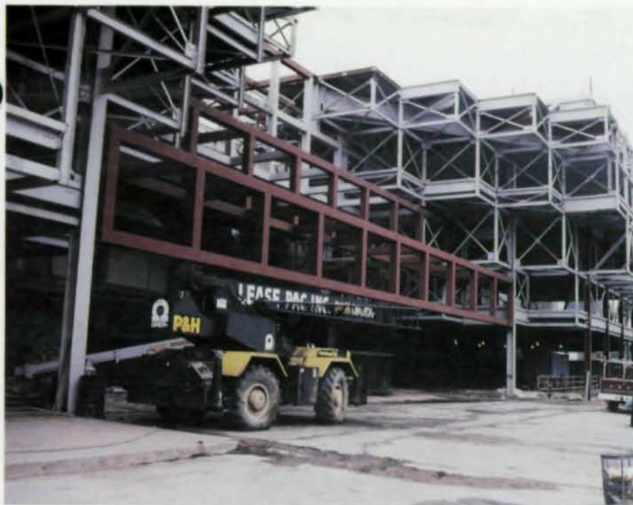
East side expansion, atrium area, with Vierendeel trusses, cantilevered facade
