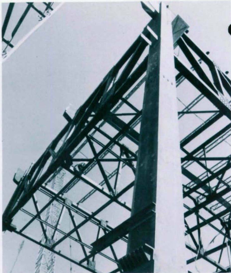
Steel box column (30x30 in.), north expansion
