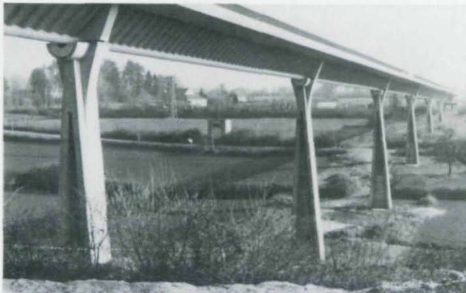
Maupre Viaduct after completion
