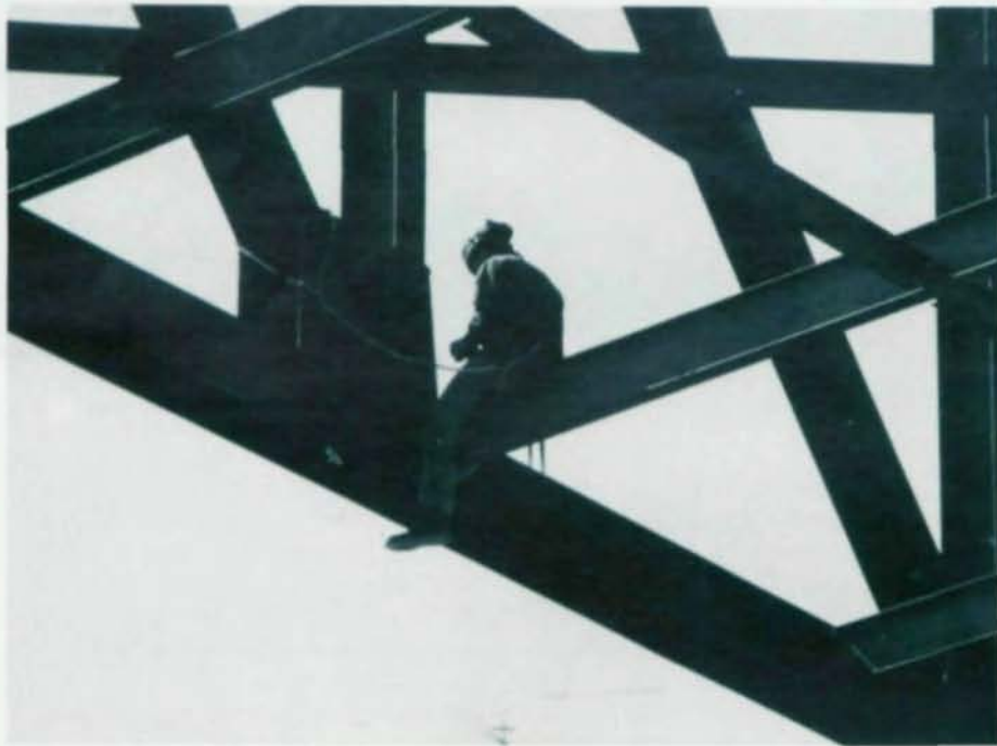
Ironworker on wide-flange truss, north expansion
