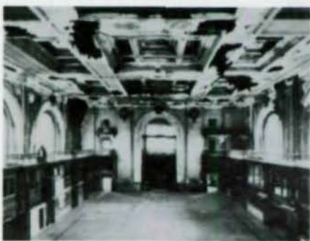
Before —interior of ravaged Union Station
