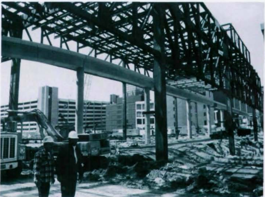
Framing over people-mover guideway, north expansion
