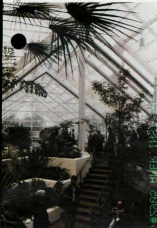
Tropical house showing six-tube connection
