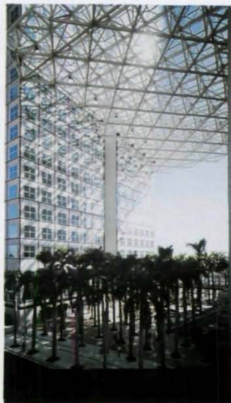
Magnificent 12-story high steel space frame, painted white, covers pedestrian plaza.
