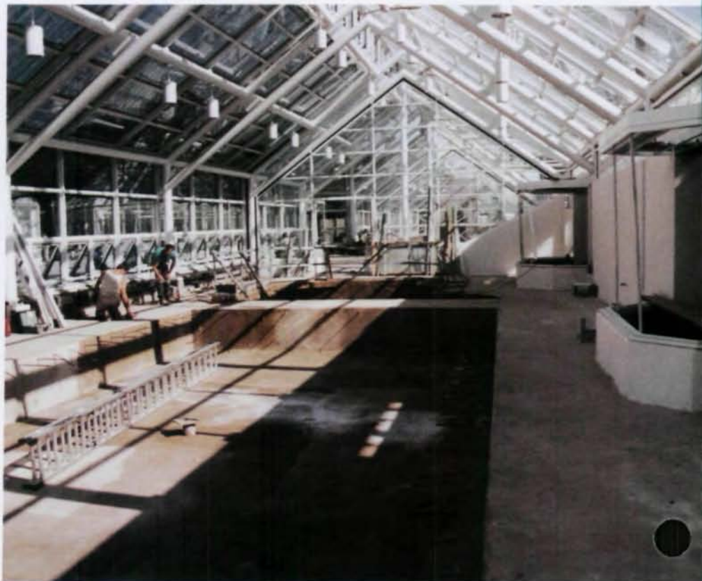
Typical greenhouse roof framing
