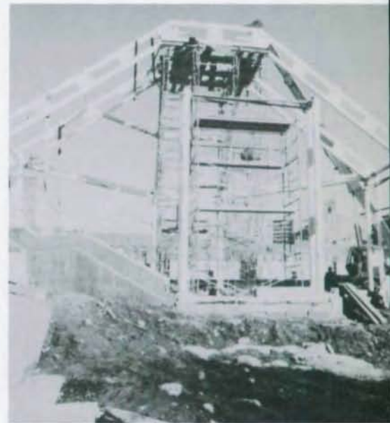
Erection complete on one cross space-truss frame.
