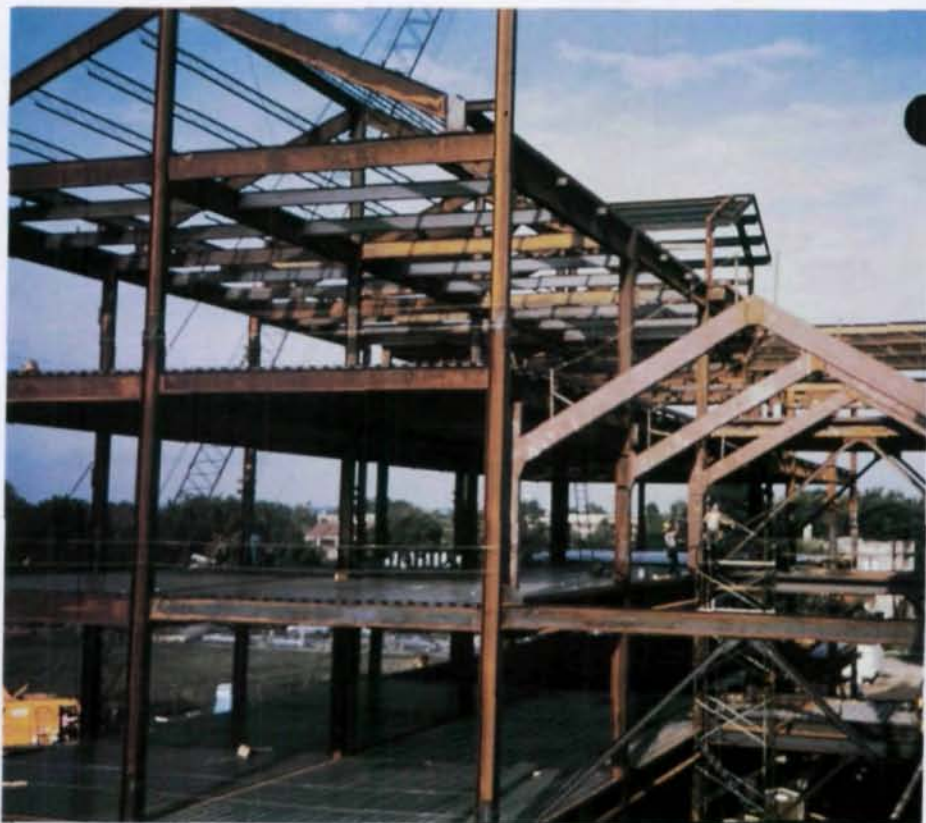
Steel construction of atrium roof members
