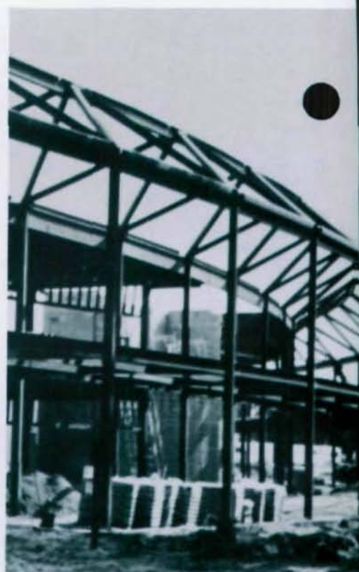
Steel members frame distinctive curved circulation spine
