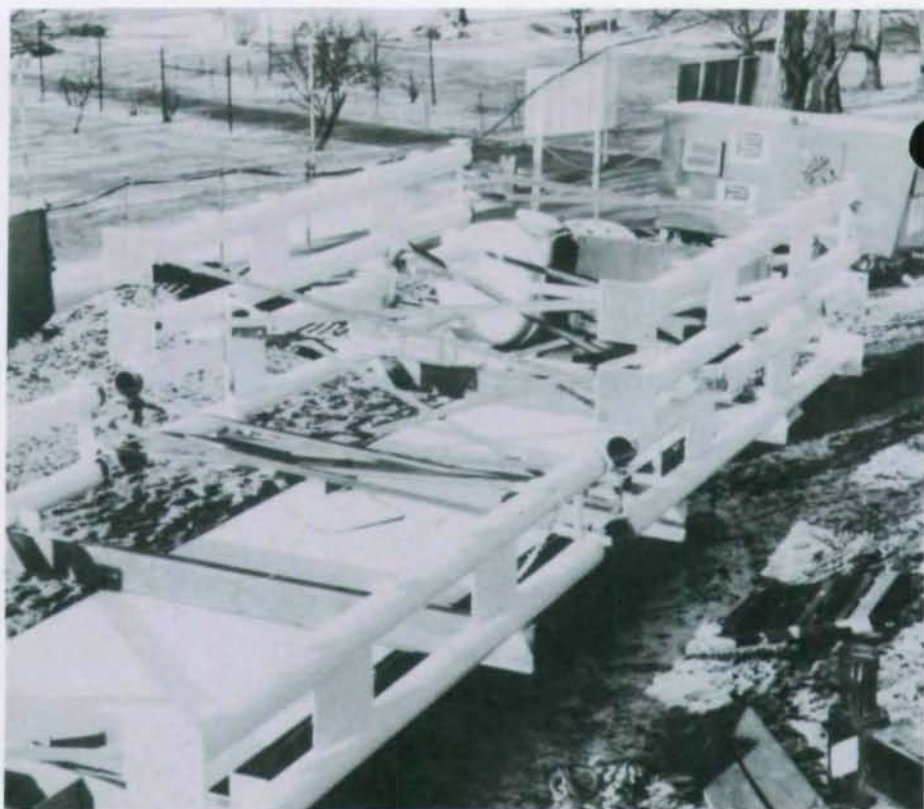
Prefabricated space trusses as they arrive on site.
