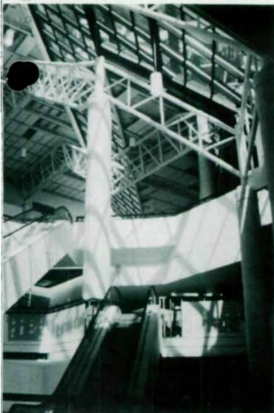
Interior view of stair-step trusses in airport atrium
