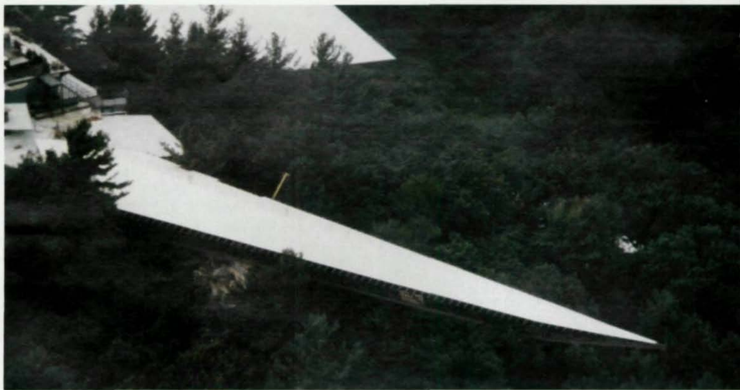
Air view of Infinity Room. Rock outcrop (c.) supports 140-ft cantilever over valley.
