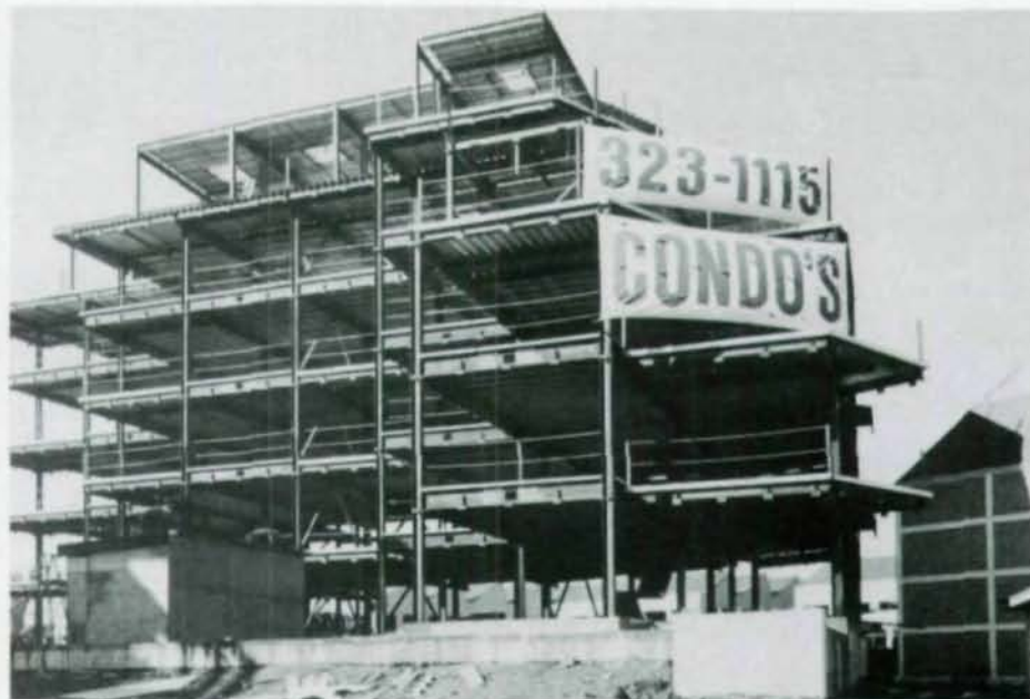
Terraced steel frame
