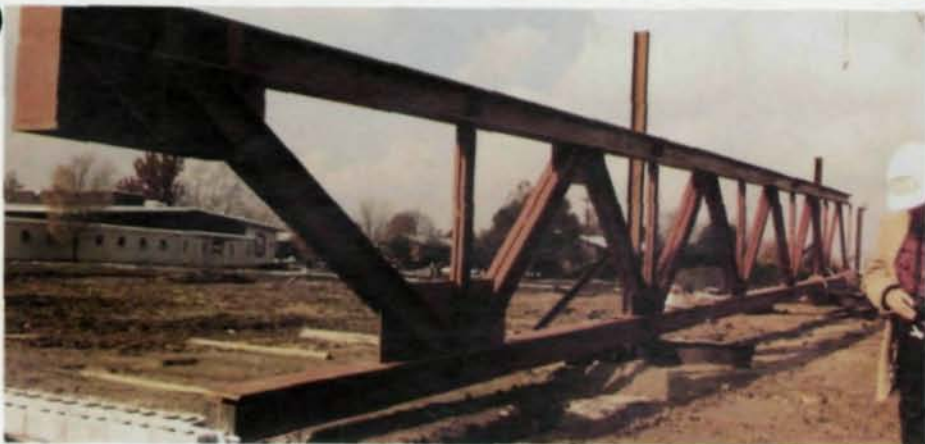
Horizontal truss element of typical bent, supported by temporary erection frames
