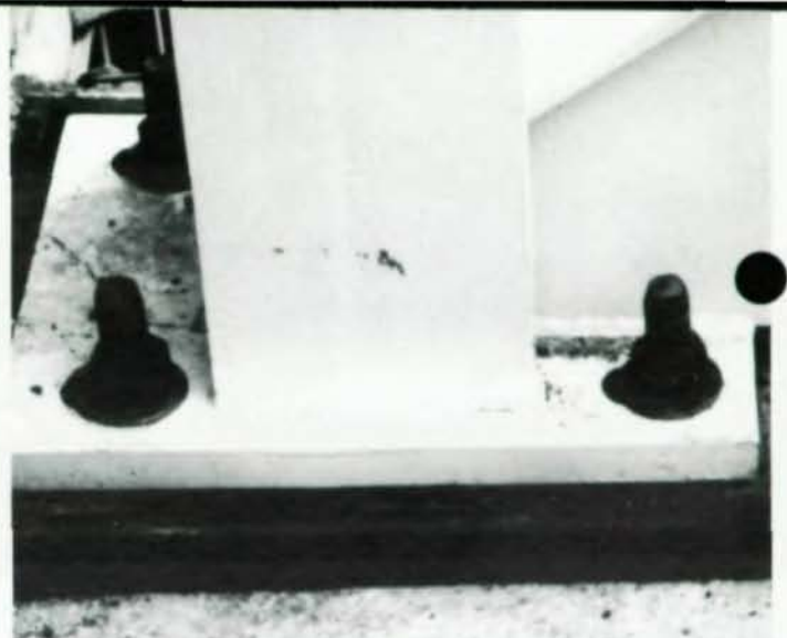
Closeup of truss support
