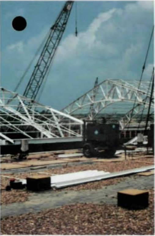
Roof scene shows how trusses are erected.
