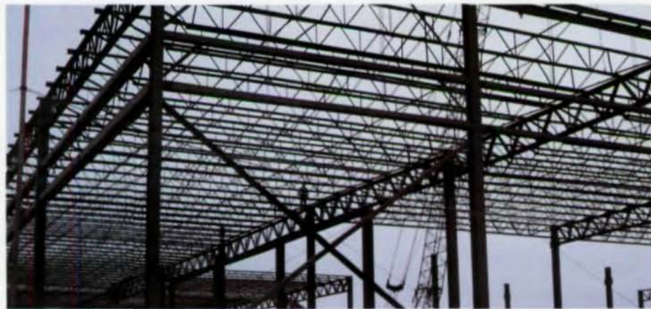
Structural steel framing provides 37 ft of ceiling clearance for parts storage.
