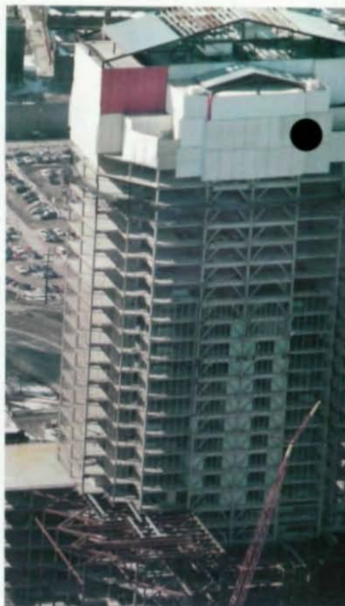
Aerial of steel-framed Three Nationwide Plaza. Fred Schaal/Aerographics photo. Below, North atrium exterior under construction.
