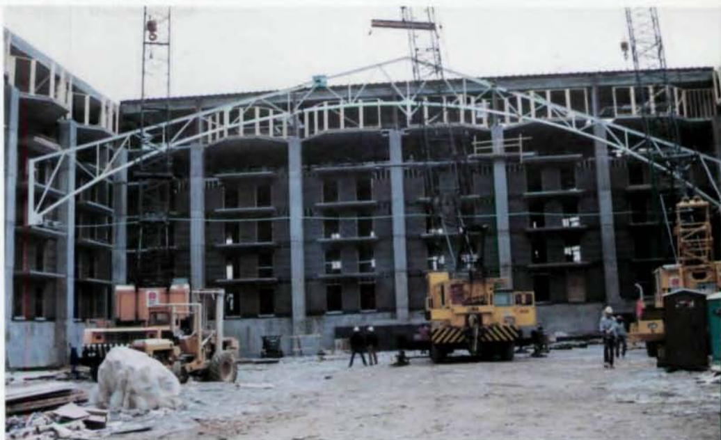
Truss erection used three cranes.
