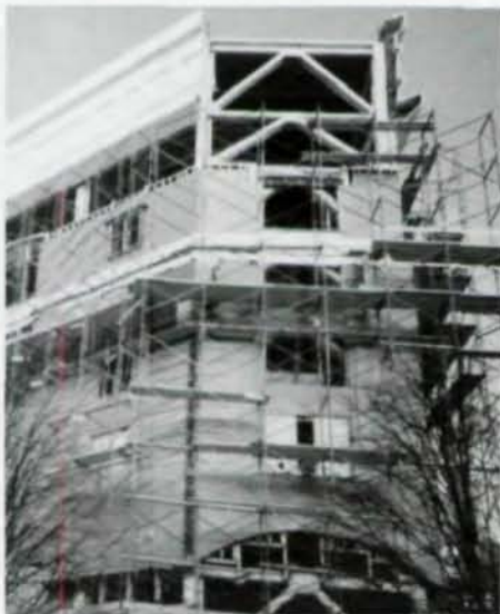
Cornice panel supported on steel framing.
