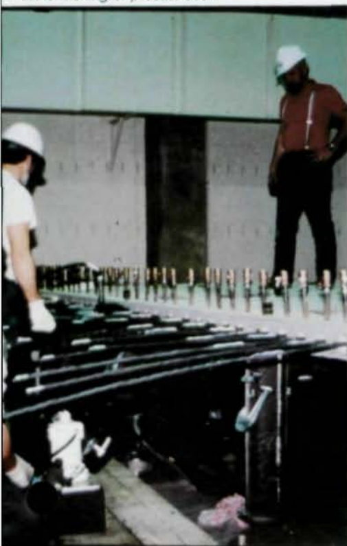
Post-tensioning of precast deck
