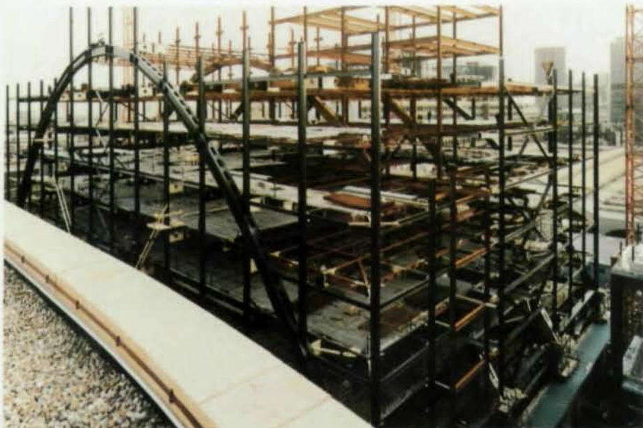
Unique structure required high degree of dimensional control in steel fabrication.
