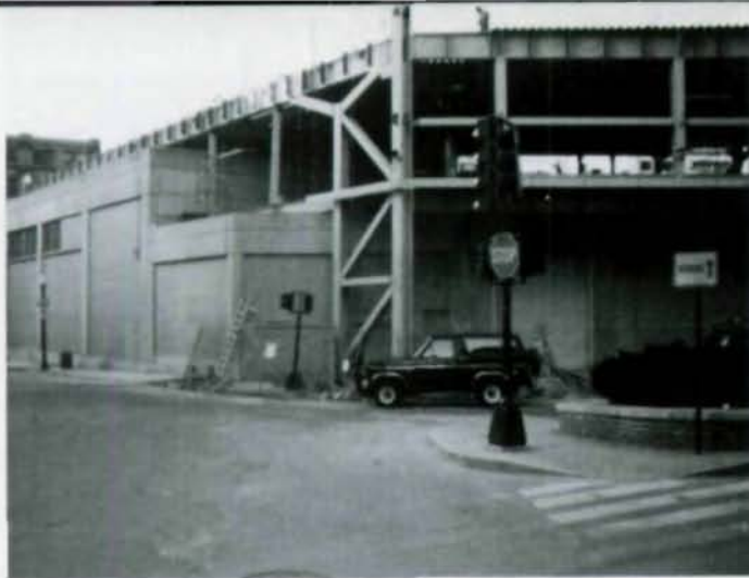
First part of truss erected (l.). . . and completed truss spans existing station.
