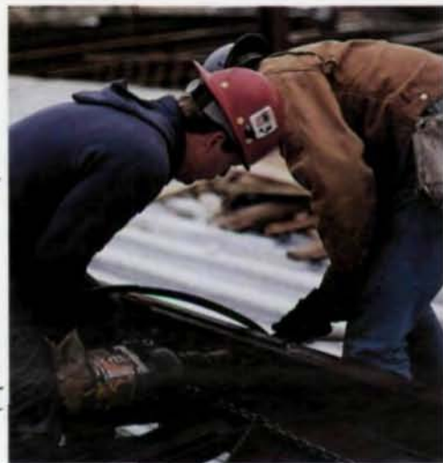
Joist sections are easily assembled on site.
