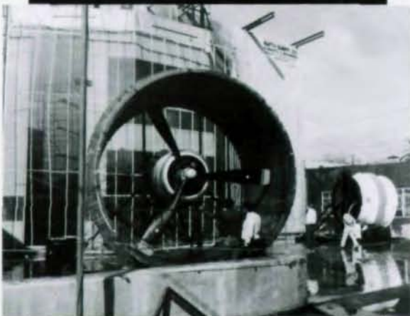
Wilshire/Westwood, Los Angeles Granite and Aluminum/Glass Window Wall Mockup ready for Dynamic Water Infiltration Test.
