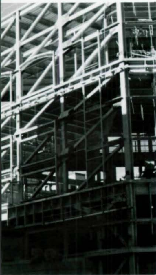
Tubular frames (top) support windows erected in front of truss. Below, opportune location for lateral bracing.
