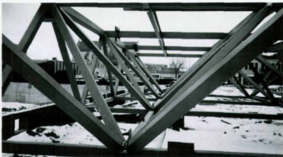
Space frames in assembly fixture
