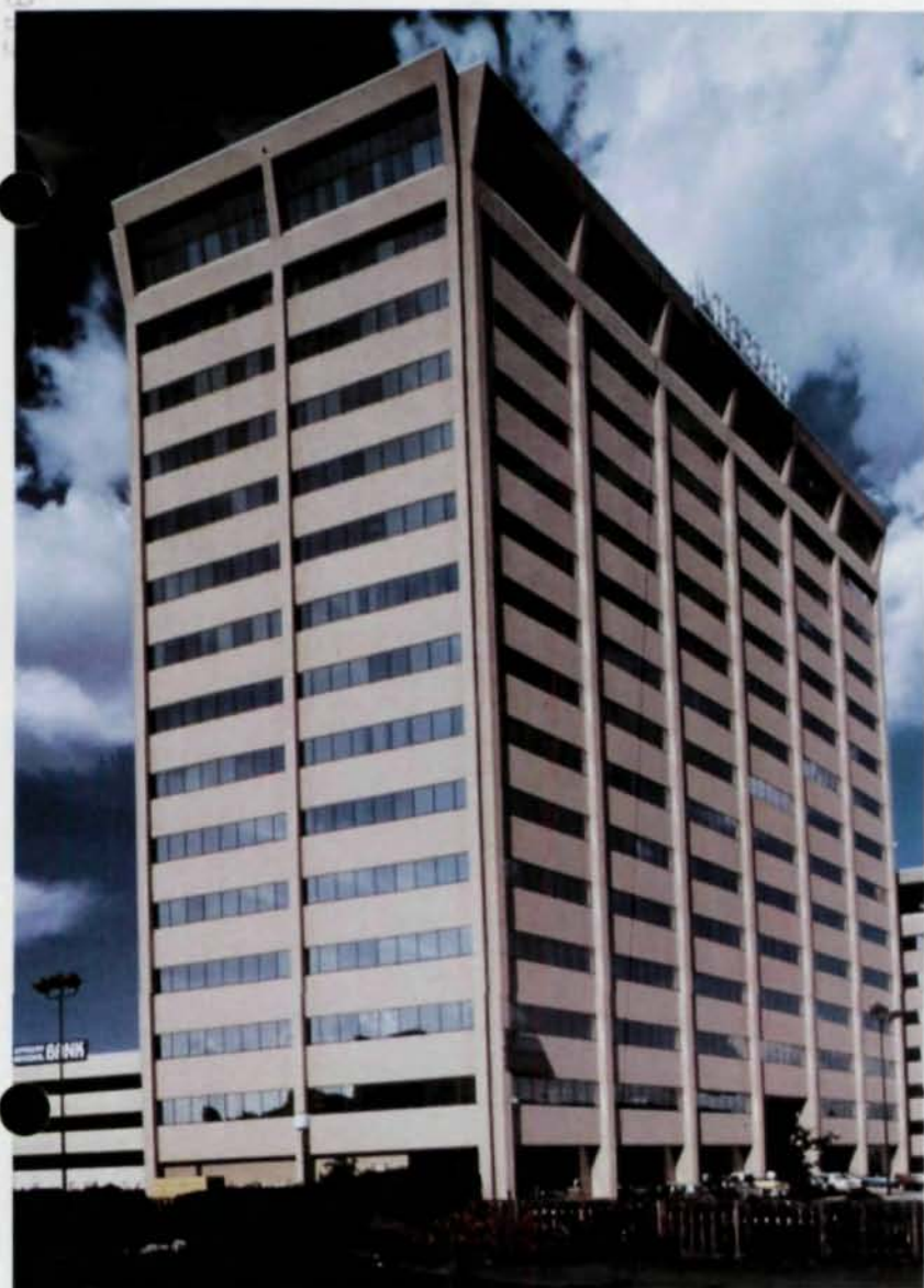
Building before extensive skin remodeling
