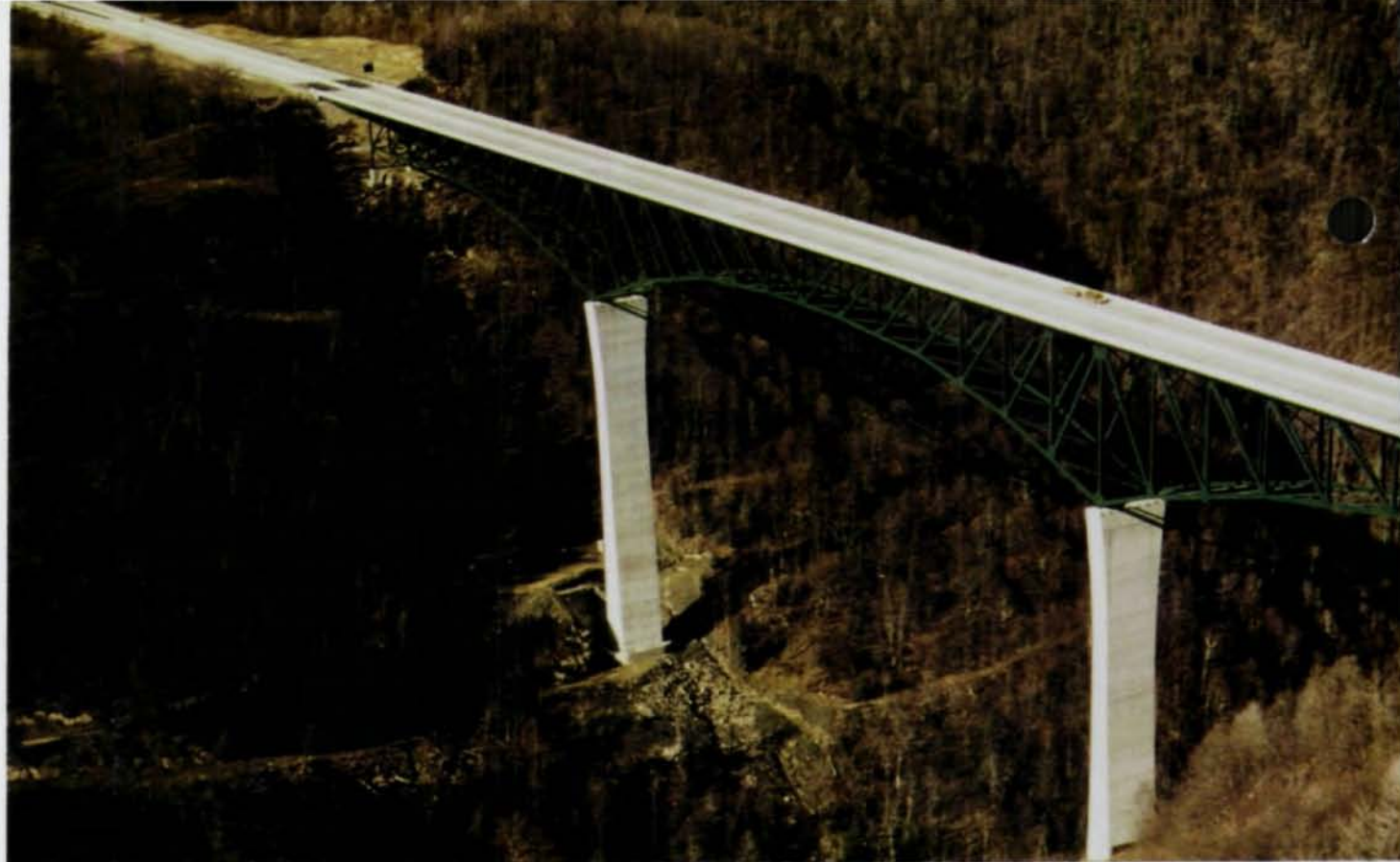
Dramatic steel span over deep gorge near Beckley, W. Va.
