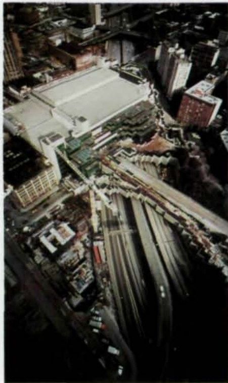
Traffic moves at regular pace despite massive construction overhead.
