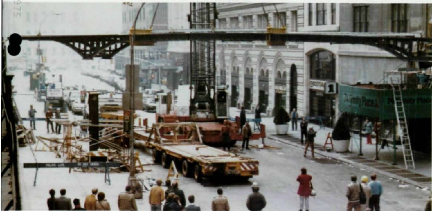
Bridge swings into place overnight to eliminate any traffic jams.
