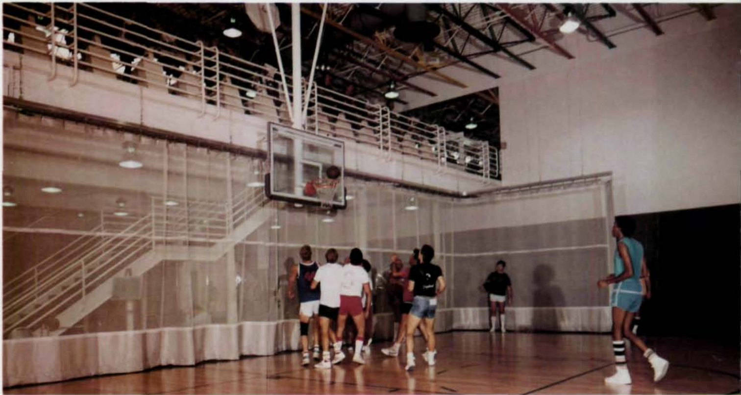
A "weighty" problem was solved by using steel framing on sports club atop Bellevue parking deck.
