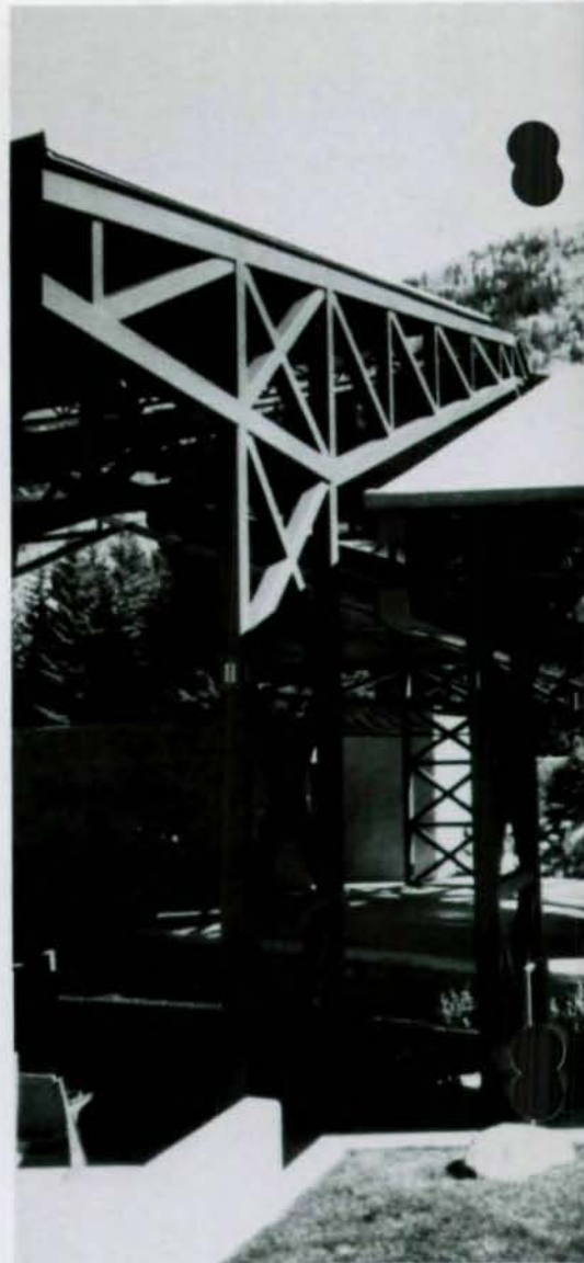
Amphitheater is central element of 23-acre Ford Park. Natural land bench shaped site. Exposed steel structure is the architecture. Free-standing space trusses are structurally sound without need for lateral resistance of roof decks (1. and above).
