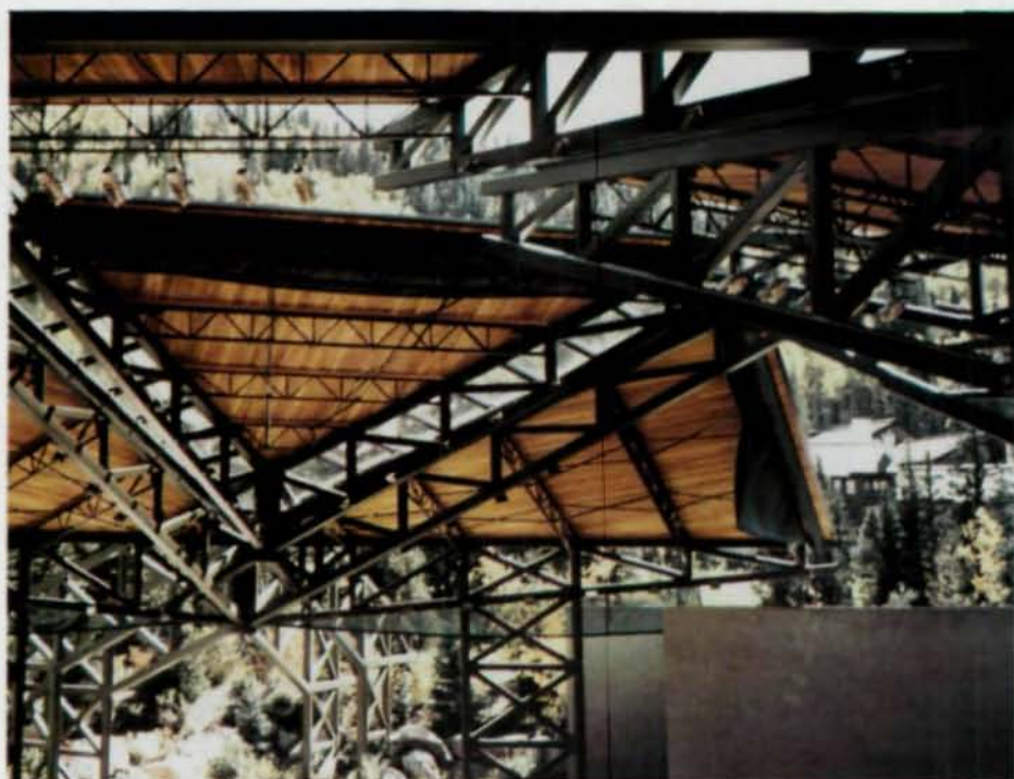
Structure is architecture at amphitheater, where space is defined by tubular steel trusses that are light and sculptured and lend feeling of spaciousness.
