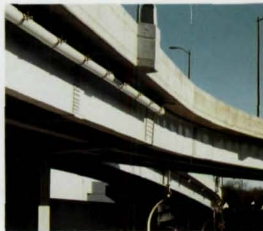
Elevation looking southeast, with Ramp A in background.
