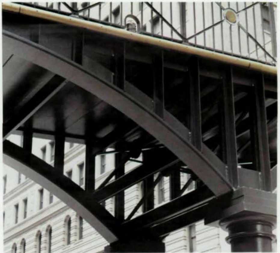
Closeup of bridge shows intricate detailing of structural steel and railing.
