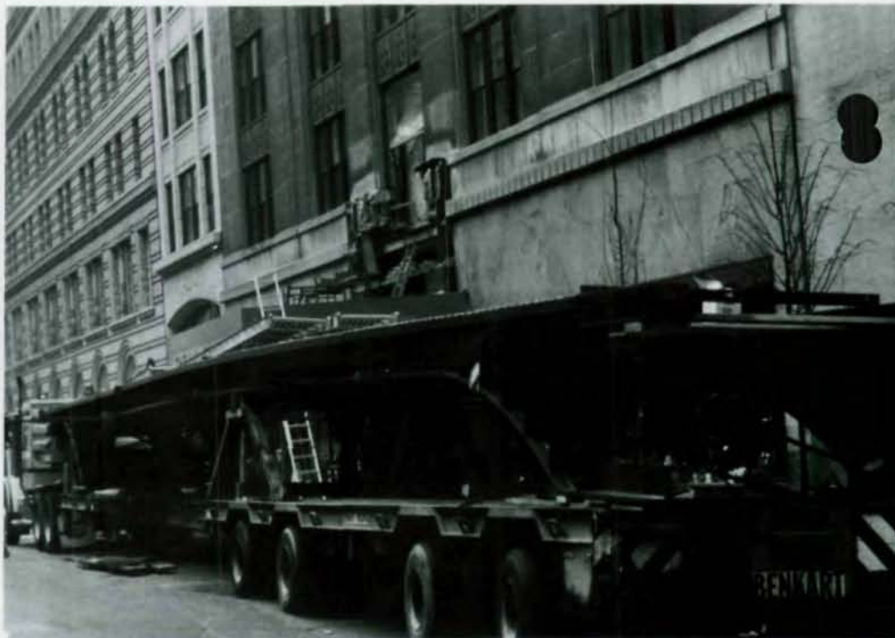
Trinity Bridge transported to busy Manhattan street in one piece on special trailer.
