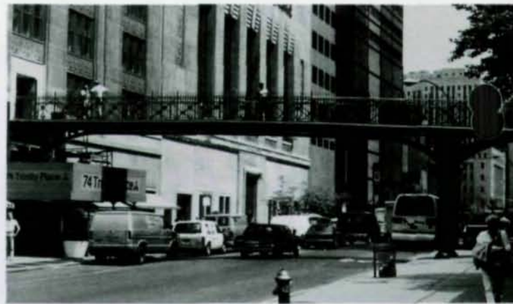
Finished steel bridge joins Trinity Church with Trinity Place across busy thoroughfare.
