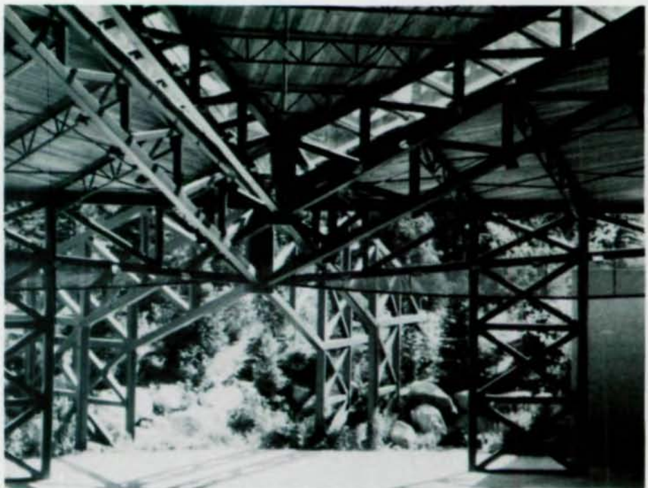
Two hexagon tube-plate connections at intersection of several truss frames.
