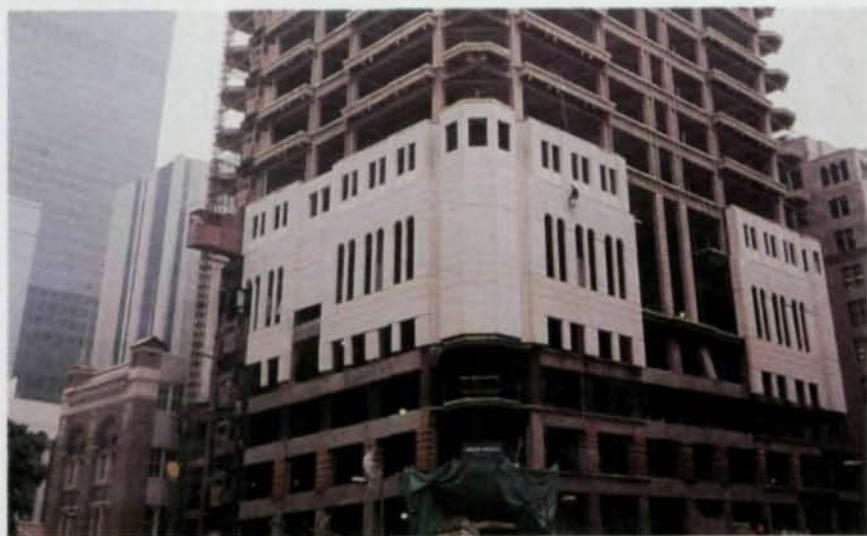
The architect of the Home Savings Tower in Los Angeles chose to design the building in the French Chateau Style to help recapture the positive feeling created by the architecture of the past. The project's structural system was complicated by the need to slope the steel columns at the sixth (see below) and the 24th floors. Construction photography by Annette Del Zoppo.
