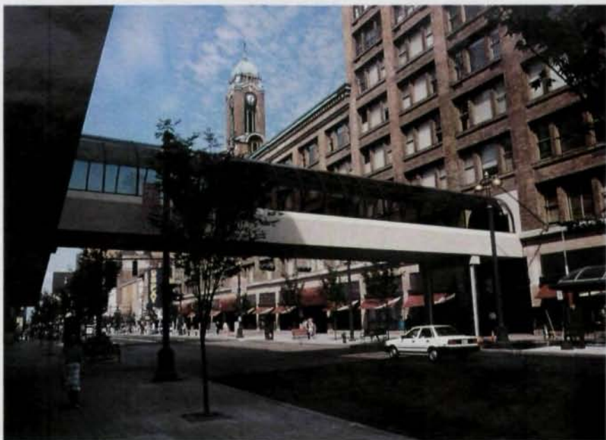
Construction of Rochester, N.Y.'s newest pedestrian skyway was facilitated by the use of steel. Because steel can be readily spliced, the 96'-8" span was broken into two pieces, facilitating transportation and erection of the girders.
