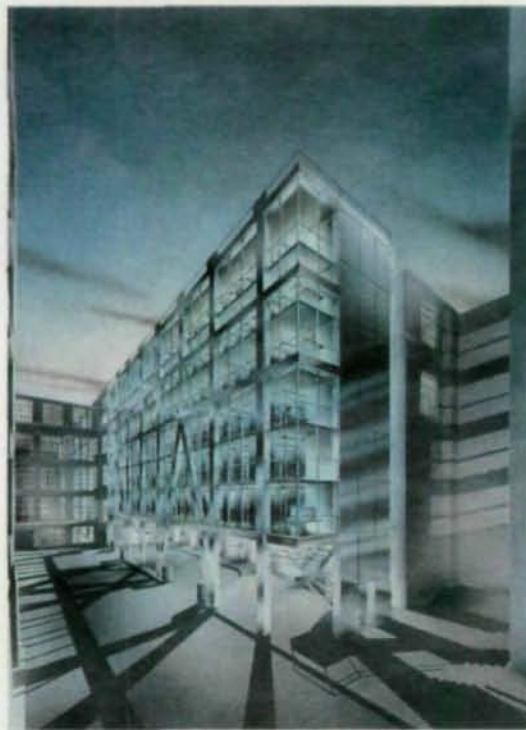
The steel frame for the new MIT Library of Architecture (opposite and left) serves a dual purpose: form and function. Because the perimeter columns are 15'-on-center, there was inadequate room for trucks to enter and turn around beneath the library. To accommodate the trucks, two of the columns were split at the fourth level and form an "A" shape. Photography by Curt Berner. Rendering by Don Paine.
