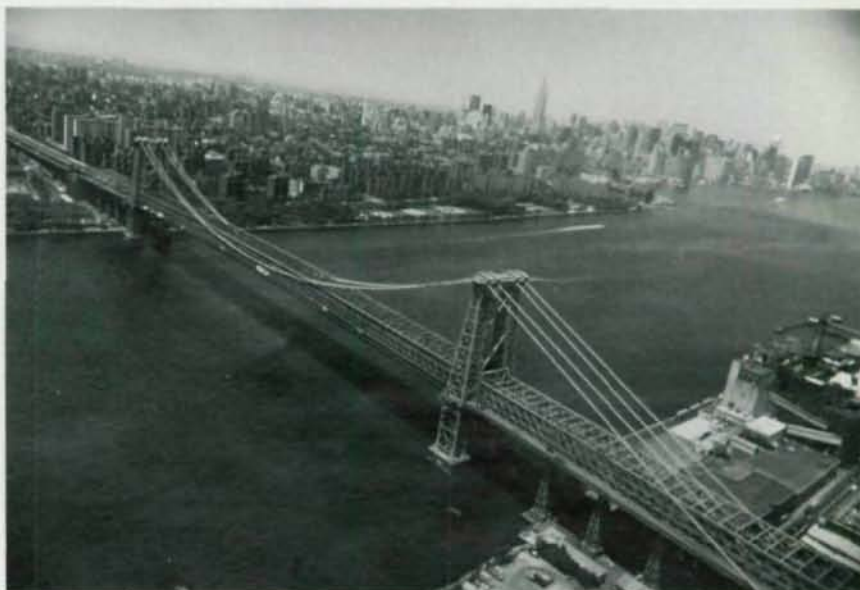
The Williamsburg Bridge, which opened in 1903, is scheduled to undergo a $400 million rehabilitation—the largest in New York's history—to be completed in 1998.
