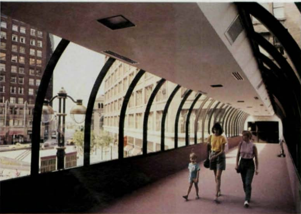
A new pedestrian walkway in Rochester, N.Y., hooked two large department stores into the city's elaborate latticework of skyways. The 96'-8" pedestrian bridge was designed in steel after it was determined that a concrete bridge would not be completed on time or on budget.
