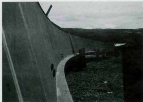
Pictured at left is a fabricated tub ready for spot blasting and the application of a full primer coat. The rust stain spreading from the exposed weld bead does not inhibit the adhesion or corrosion protection provided by the primers.
