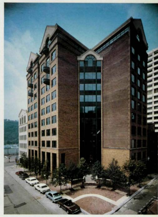
A 28,845-sq.-ft. addition was constructed as part of the renovation of the former Shields Rubber Co. Warehouse into a modern office building. The use of a lightweight steel frame was essential to match the floor heights of the existing building and to provide the desired 35' on center bay spacing. Construction photography by Fred P. Kenderson; finished photography by Maureen Wikiera.
