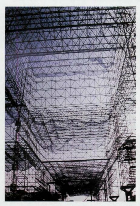
Pictured above is the magnificent Jacob K. Javits Convention center in New York, which uses HSS to create a memorable main hall to a mostly undergound convention facililty. On the opposite page is the United Airlines Terminal at O'Hare Airport in Chicago, which recalls the glorious train stations of an earlier age.
