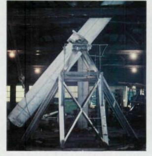
Crossbracing (above) was installed on each end of the span to tie each pair of trusses together.
