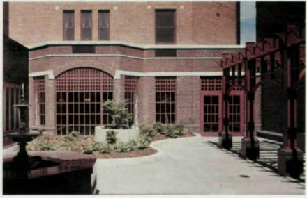
The large setbacks, combined with the decorative exposed steel, breaks up Canterbury Place's huge mass and allows it to better meld with the surrounding community. Exposed steel is used in a variety of ways on the project, including the prote cochere/entrance, trellised walkway, upper level wind and sunscreens, and for the steel-framed windows.
