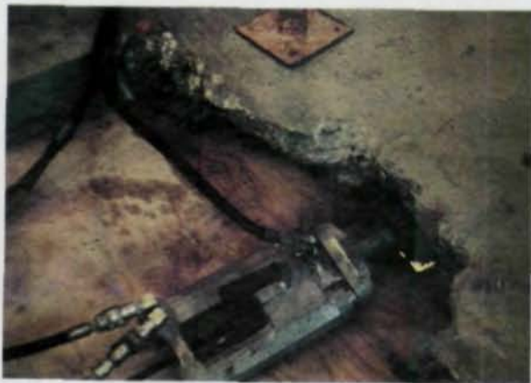
Supporting the new office building was extremely complex because the parking deck was post-tensioned concrete. The tensioning rods had to be located and a post tension jacking device was used to reset the cable at each end of the hole cut for the new concrete piers.
