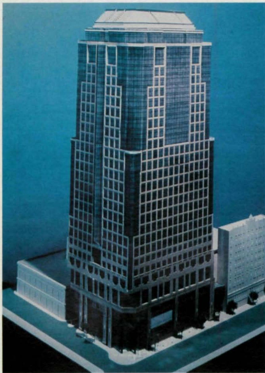
The 31-story Walnut Building in Kansas City, which is still under construction, was built on top of an existing six-story parking garage.
