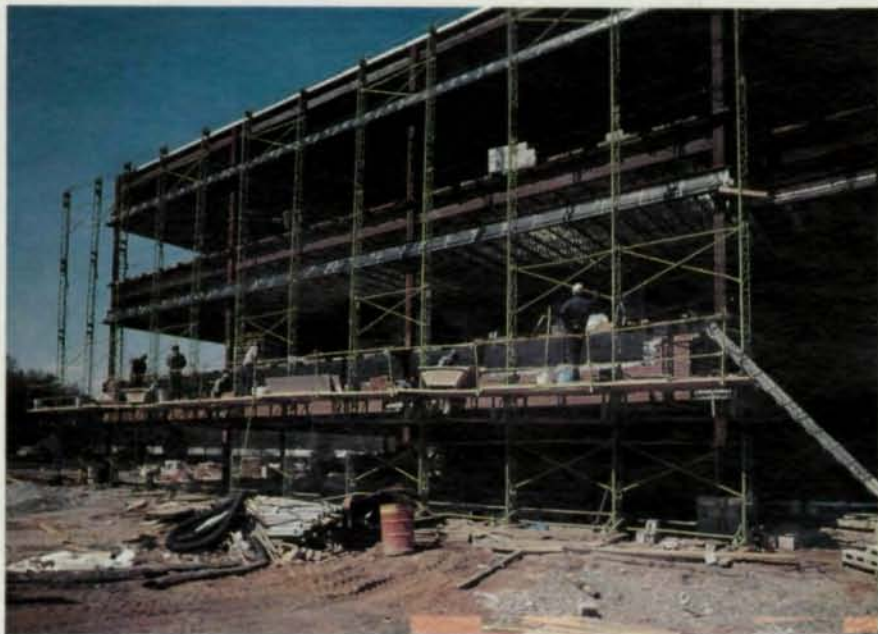
Because the owner had a preference for avoiding a structural steel stud system to support the masonry cladding, the engineers designed a block and brick veneer system. The projected curtainwall, which did not effect the project cost, is supported by lintel spandrels. Photographs courtesy of Bass Construction
