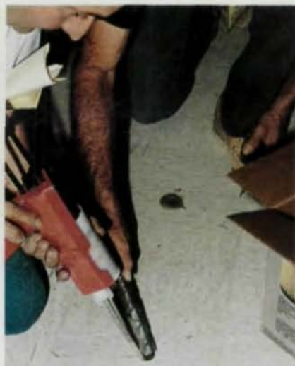
New steel studs were welded to the steel girders to provide composite strength (left), while high strength non-shrink grout was used to insure adequate bonding (above left). The contractor installed new steel dowels to tie the two layers of concrete together without interrupting any hospital functions (above).
