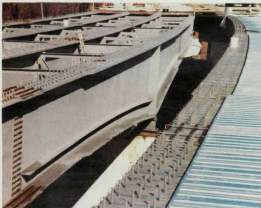
Based on preliminary investigation and a desire to minimize deck expansion joints, the bridge spans selected are nominally 150' in length and are arranged in five-span continuous units of 750'. A three-span continuous haunched unit (above) with a center span of 215' is located over the Kanawha Canal.
