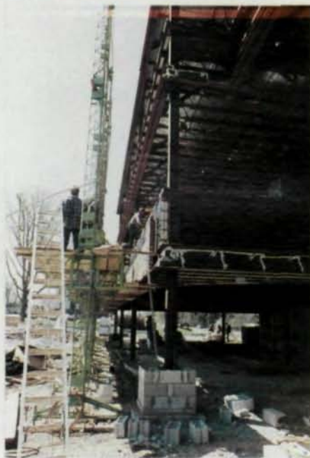
Because the owner had a preference for avoiding a structural steel stud system to support the masonry cladding, the engineers designed a block and brick veneer system. The projected curtainwall, which did not effect the project cost, is supported by lintel spandrels. Photographs courtesy of Bass Construction
