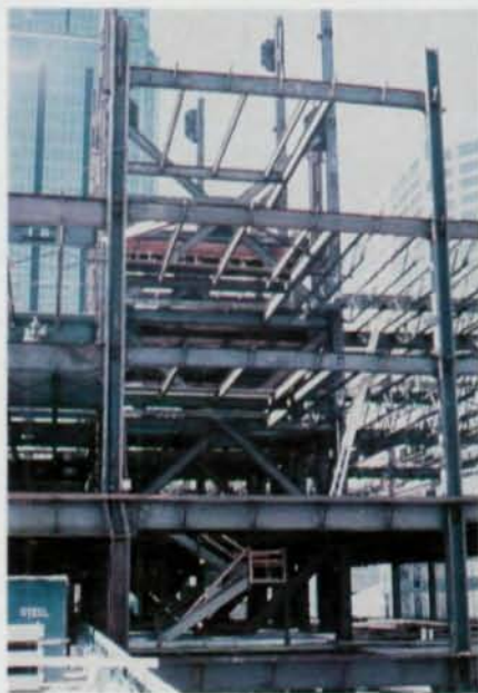
The structure is partially stabilized with braced frames around the elevator core. In the north/south direction, X-bracing was used to take advantage of the economies inherent in a two-story high frame. The bracing consists of double channel members back-to-back, connected through their webs to gusset plates shop welded to columns and struts.
