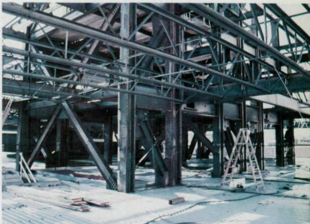
The structure is partially stabilized with braced frames around the elevator core. In the north/south direction, X-bracing was used to take advantage of the economies inherent in a two-story high frame. The bracing consists of double channel members back-to-back, connected through their webs to gusset plates shop welded to columns and struts.
