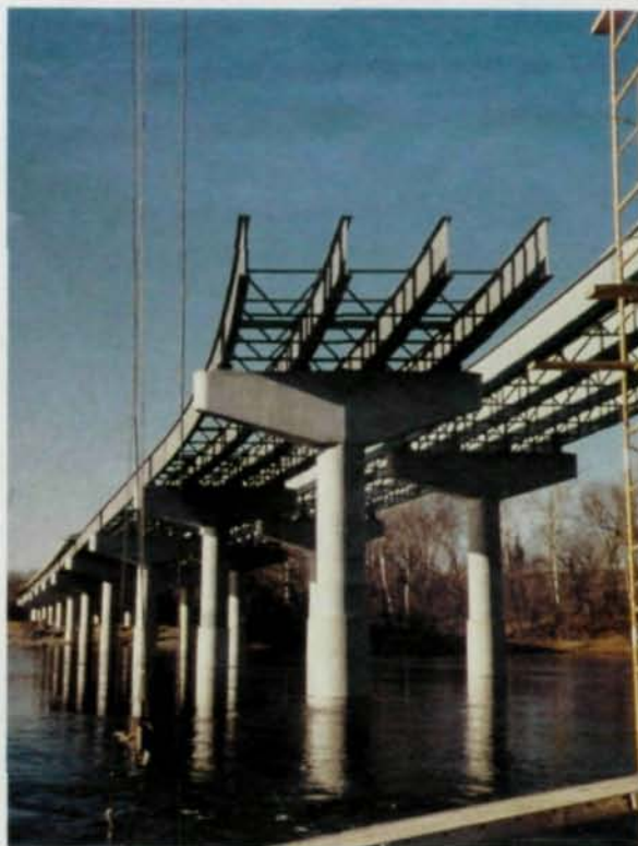
Based on preliminary investigation and a desire to minimize deck expansion joints, the bridge spans selected are nominally 150' in length and are arranged in five-span continuous units of 750'. A three-span continuous haunched unit (above) with a center span of 215' is located over the Kanawha Canal.
