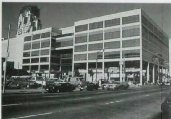
Surprisingly, a relatively new five-story concrete office building came through the earthquake unscathed. Upon closer inspection, it becomes apparent that damage was most likely prevented by reinforcing the soft first story with steel-braced frames.
