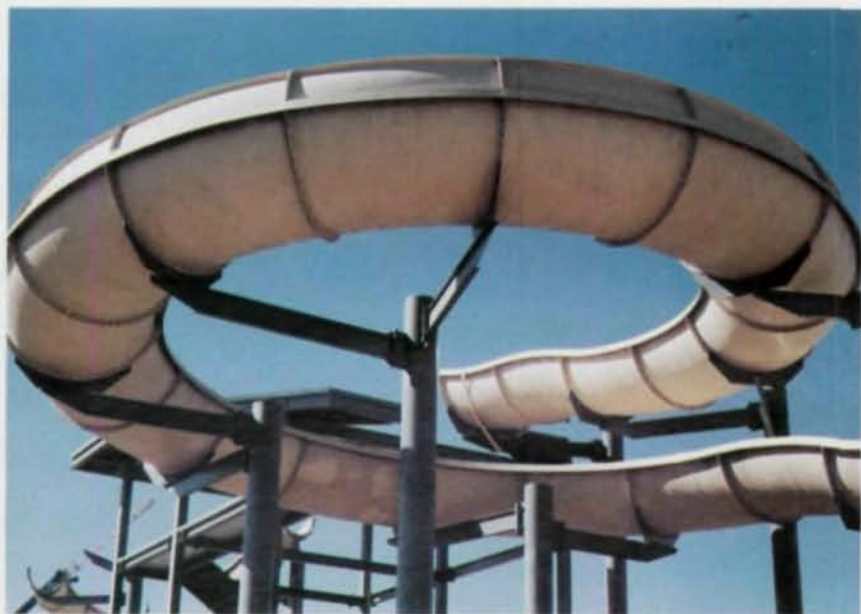
The supporting arms on the giant "Twister" at Wild Waters in Sparks, Nev., are WF sections, though on other projects they are usually structural tubes.
