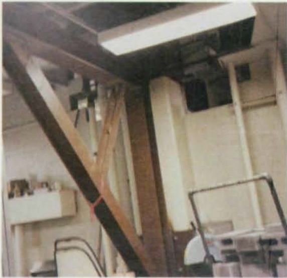
The most complicated aspect of the project was incorporating a bracing system in the new and existing structures to resist wind and seismic forces. However, the number of locations and the configuration of the bracing was limited because it was crucial that the floor not be disturbed or limited. A scheme of eccentric compression bracing along with inverted "V" bracing was used to avoid mechanical runs, doors, and windows. Pictured above is a steel brace placed in the existing building against the concrete frame.
