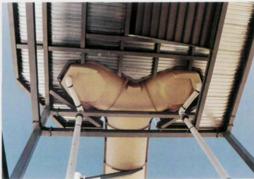
Pictured above is the connection between the stair tower and the slide of a giant twister at Wild Waters in Sparks, Nev.
