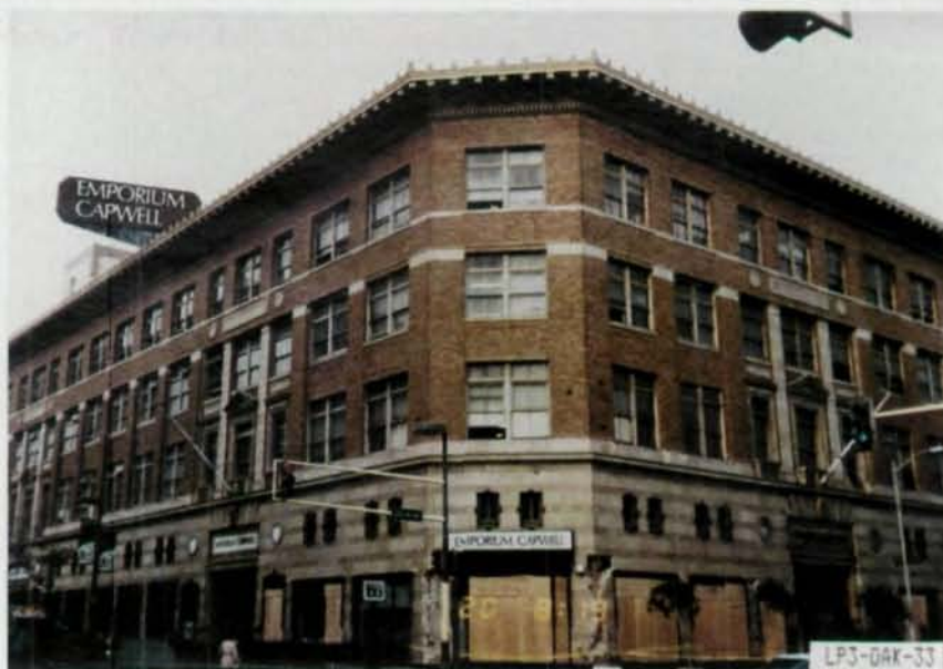
One of the more severely damaged steel-frame structures in Oakland was the Emporium-Capwell Store, shown above and at left just following the Loma Prieta Earthquake in 1989. Extensive damage occurred to hollow clay tile brick masonry and terra-cotta trim on the building. The steel frame, however, was undamaged.
