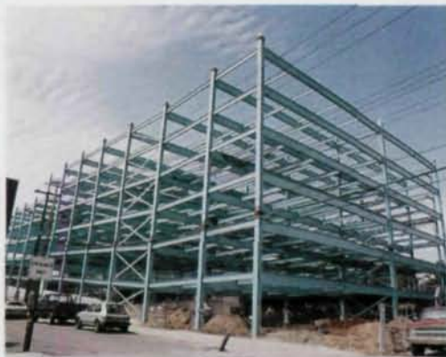
Albert Ave. Parking Structure, East Landing, MI
