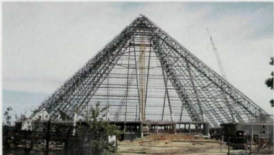
The Pyramid Arena in Memphis is a unique steel framed structure. Joists were used as part of the support system for the skin of the building.
