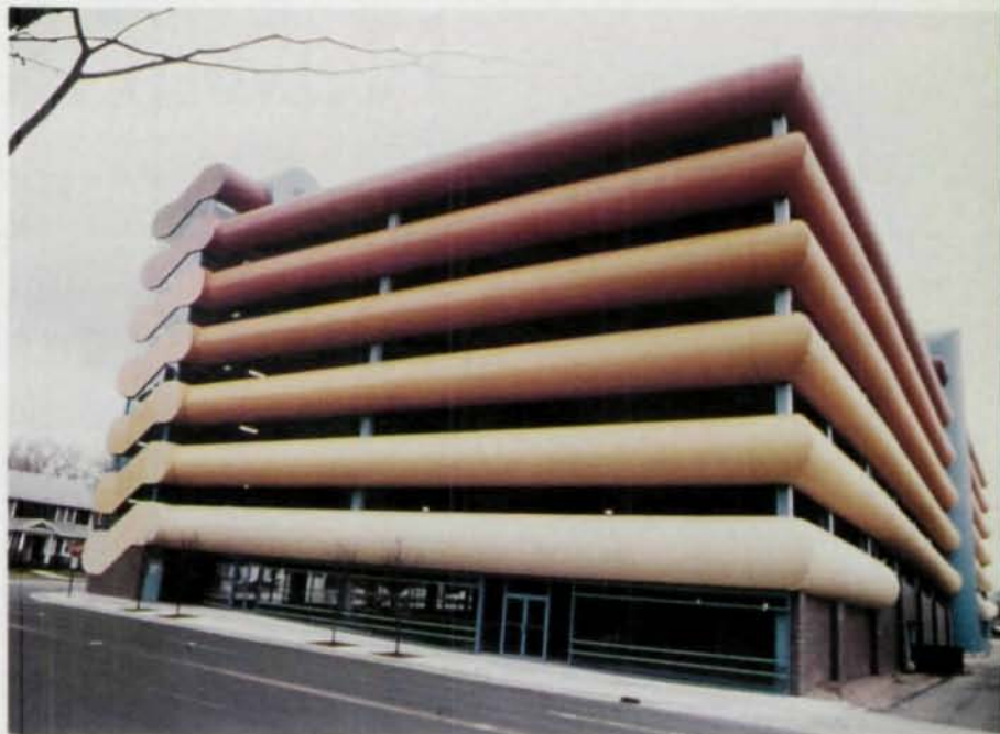
The metal panels on the exterior of the garage are made of corrugated steel. The colors were chosen to complement the colors found on neighboring structures.
