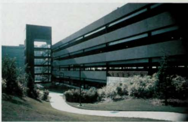
Shown at top is a detail of the barrier elements at the Becton Dickinson Parking Facility. Pictured above is University of Massachusetts Medical Center garage in Worcester. The medical center garage provides 1,498 spaces on six levels for just over $8.5 million.
