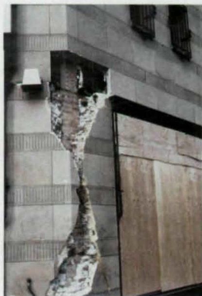
One of the more severely damaged steel-frame structures in Oakland was the Emporium-Capwell Store, shown above and at left just following the Loma Prieta Earthquake in 1989. Extensive damage occurred to hollow clay tile brick masonry and terra-cotta trim on the building. The steel frame, however, was undamaged.
