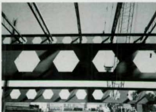
These castellated beams weigh between 60 and 70 lbs/ft.
