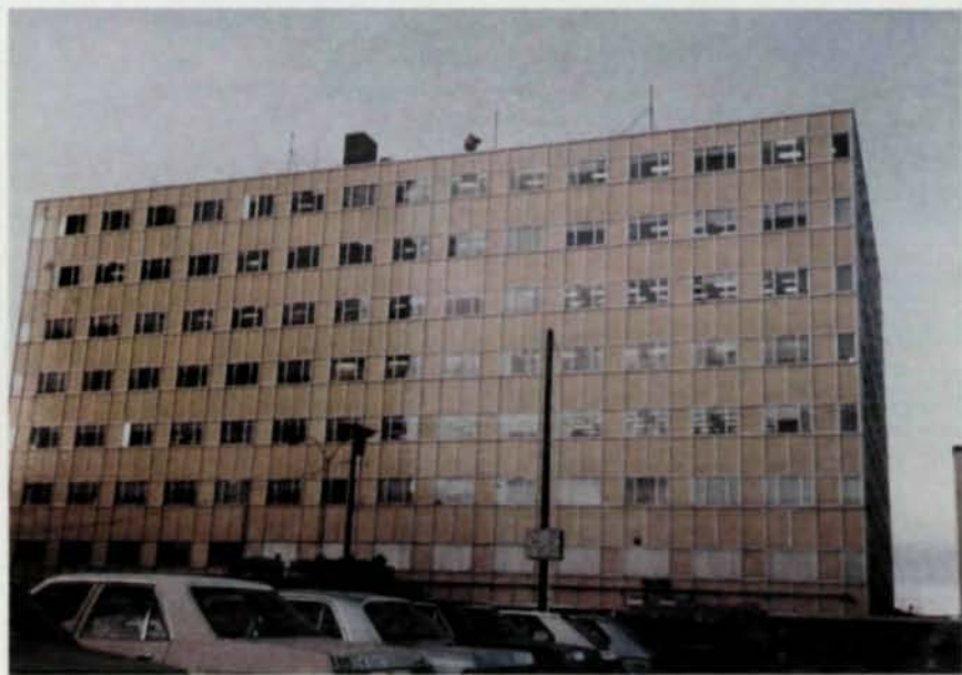
Strong ground motion during the Prince William Sound earthquake in 1964 caused the collapse of this concrete structure with masonry infill (top). In contrast, the steel-framed, eight-story Hill Building is still standing 26 years later.
