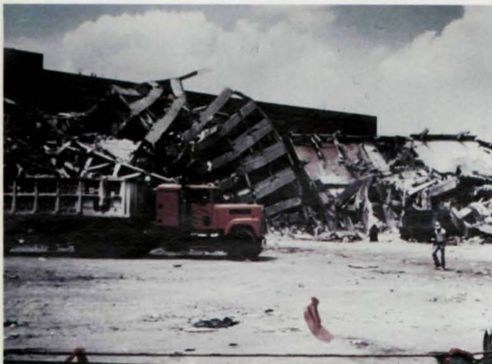
More than 300 buildings—many of them mid- and high-rise structures, collapsed during the 1985 Mexico Earthquake, which registered 8.1 on the Richter Scale.
