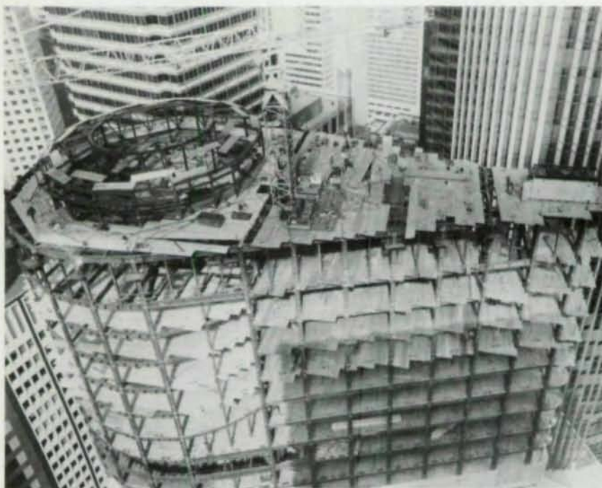
The multiple-tube design utilizes ductile, moment-resisting structural steel framing. The 18-deep columns are spaced 16' on center to maximize vision lines and reduce fabrication and erection costs. Construction photography by Edwin T. Scott
