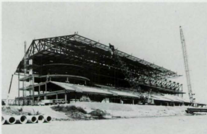
The large trusses were assembled on the ground to very tight tolerances. Safety nets were attached to the trusses with twin cables and pulled into position before the iron workers were allowed onto the trusses, which were erected 100' in the air.
