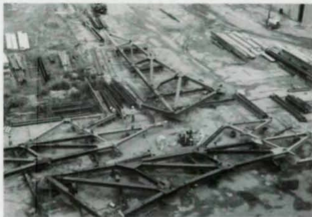
The large trusses were assembled on the ground to very tight tolerances. Safety nets were attached to the trusses with twin cables and pulled into position before the iron workers were allowed onto the trusses, which were erected 100' in the air.
