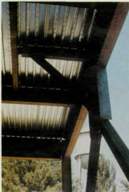
The structural system needed to be elevated and isolated from the ground in order to completely isolate the building. As a result, the building appears to "float".
