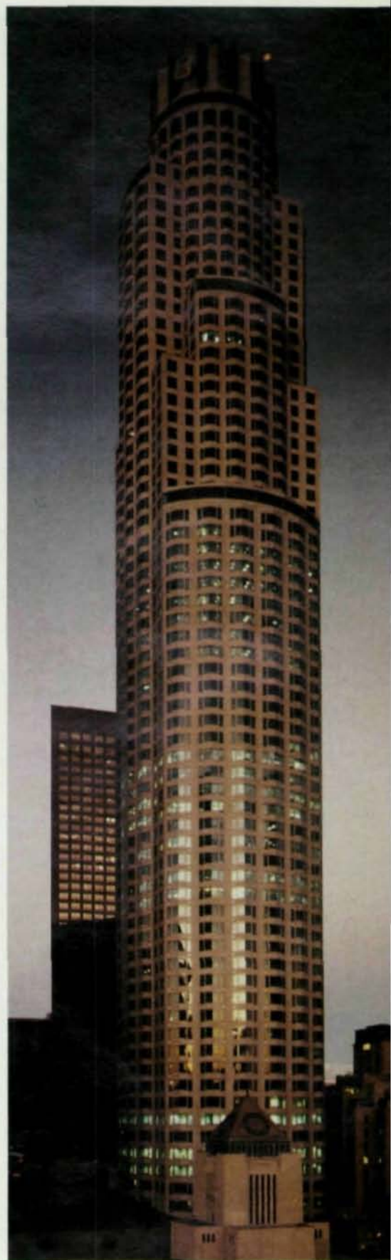
The design of 1,018'-tall First Interstate World Center in Los Angeles features an uninterrupted braced square spine, which is really a hybrid system between a dual system and a spine structure.
