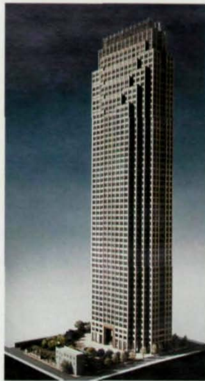
The Bell Atlantic Tower in Philadelphia is an example of a steel-framed "spine" structure with a vertical uninterrupted lateral load resisting system.
