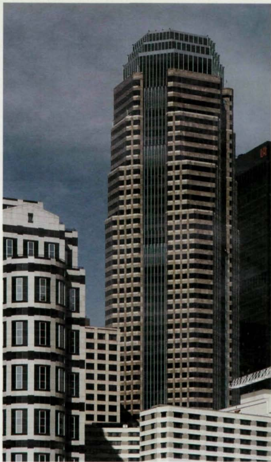
A spine structure was chosen for the Figueroa at Wilshire building in Los Angeles because it used the least amount of steel and provided an opportunity for column-free lease spaces. Photo by Erich Koyama
