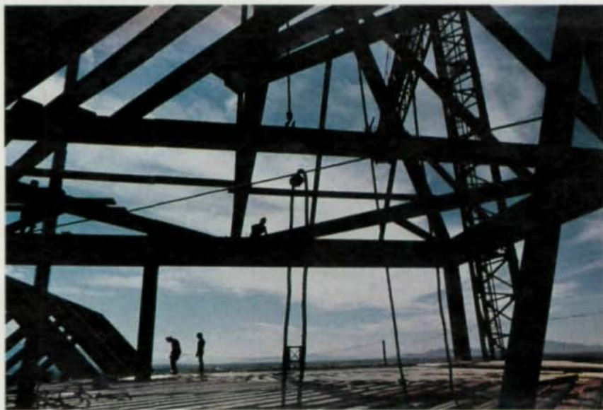
The major challenges presented by the One Utah Center project were the saw-tooth design that required an additional row of columns (left) and the pyramidal top (top and above). The center peak of the pyramid has no column, and instead functions almost as an arch. Photography by Paul Trentelman
