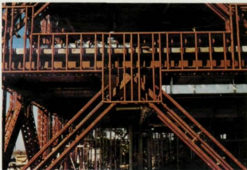
The metal cladding was carefully attached to the steel bracing to accentuate the building's structural elements and provide visual excitement.
