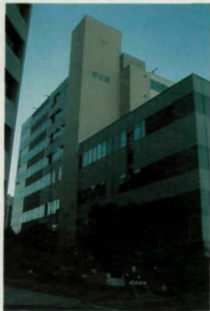
The 114,000-sq.-ft. Broadlake Plaza building in Oakland was seismically upgraded to ensure its continued survival in an earthquake-prone region.
