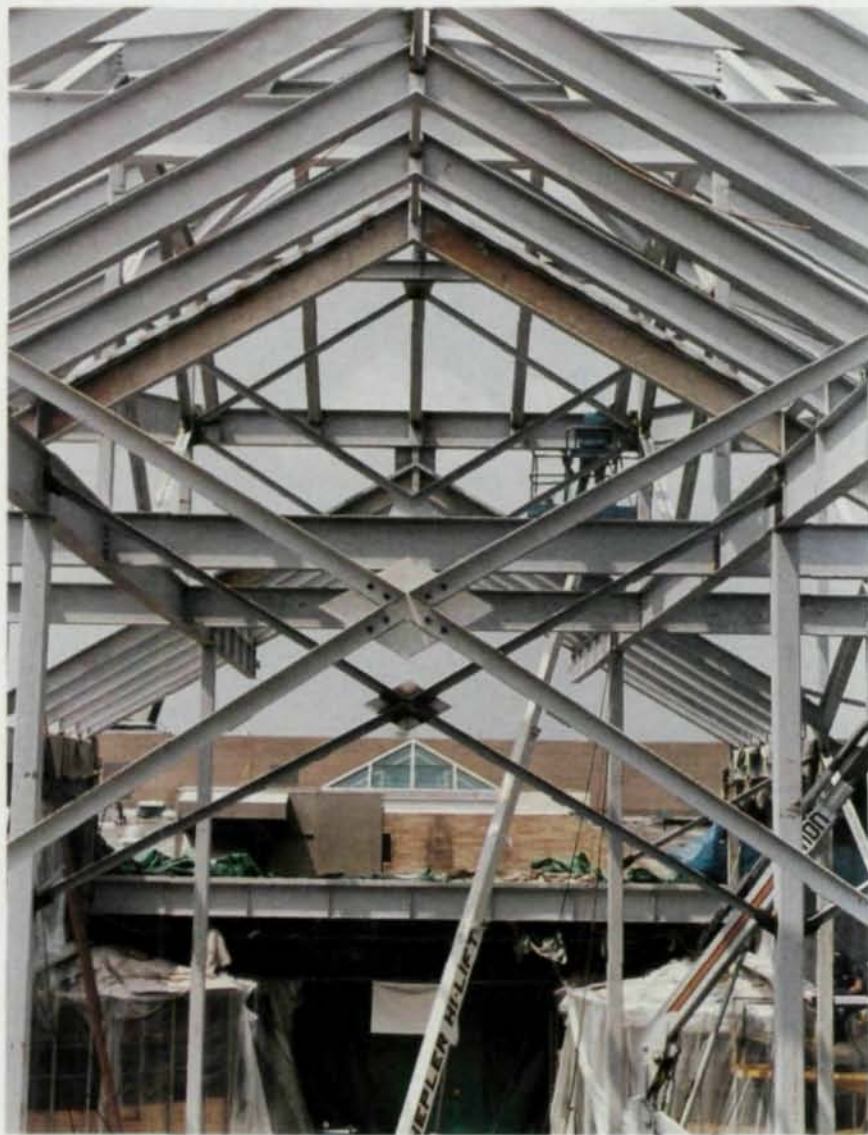
The renovated Oglethorpe Mall in Savannah, GA, utilizes exposed structural steel to create a slender, tall space and a sense of open, coastal architecture. Photo above: Henry W. Spiker; photo opposite: Gabriel Benzur
