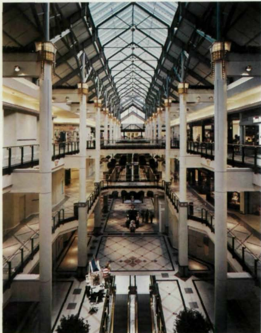
Three-story "stilt" columns support the mall structure. Garage levels were added later. Top photo by Robert E. Mikrut; photo at right by Charles Field
