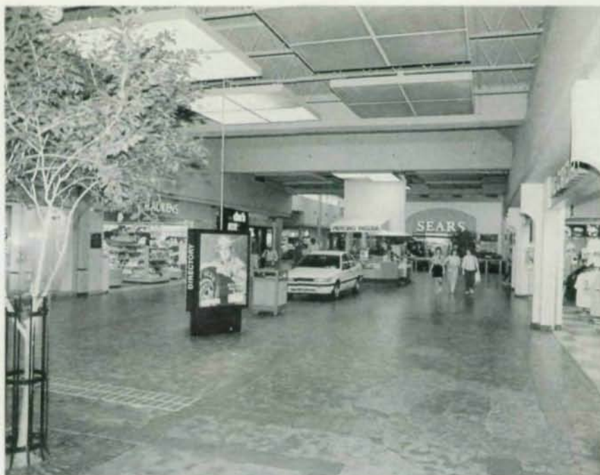
Prior to being renovated, the interior of the mall seemed gloomy, with ineffective skylights and scattered 2x4 fluorescent lights. Also, the quarry tile floor was too dark.
