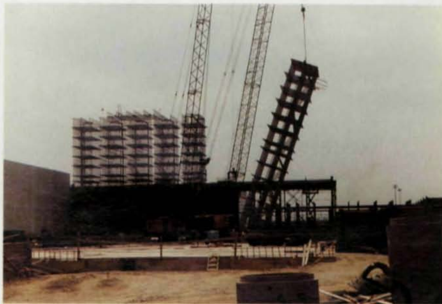
To simplify erection, the rack building is preassembled on the ground into large modules, each of which includes nine, three-post rack frames. After assembly on the ground, the 28-ton modules are tilted up and lifted into position (top photo). Lateral support is provided in the down-aisle direction with down-aisle tie angles spaced every 10' to 12', while the structure's storage shelves provide lateral support in the cross aisle direction (left photo).
