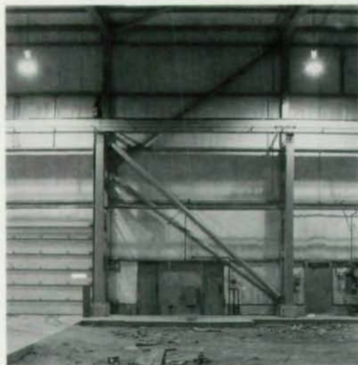
Connections are often a concern with steel tube structures. Shown above is a gusset plate welded to a column and bolted to a brace. Shown at left is the bracing for both the warehouse columns and crane girders.
