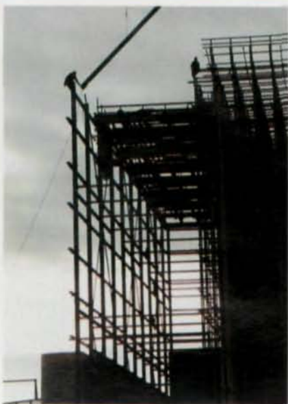
To simplify erection, the rack building is preassembled on the ground into large modules, each of which includes nine, three-post rack frames. After assembly on the ground, the 28-ton modules are tilted up and lifted into position (top photo). Lateral support is provided in the down-aisle direction with down-aisle tie angles spaced every 10' to 12', while the structure's storage shelves provide lateral support in the cross aisle direction (left photo).
