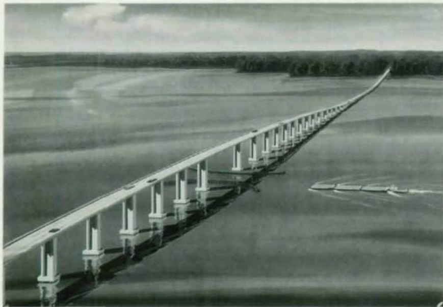
A segmental concrete bridge over the Albemarle Sound in Edenton, NC, was completed two years behind schedule and with claims totaling 61% of the original contract price.
