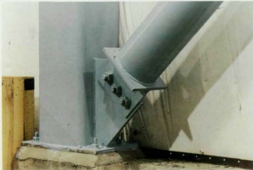
Connections are often a concern with steel tube structures. Shown above is a gusset plate welded to a column and bolted to a brace. Shown at left is the bracing for both the warehouse columns and crane girders.
