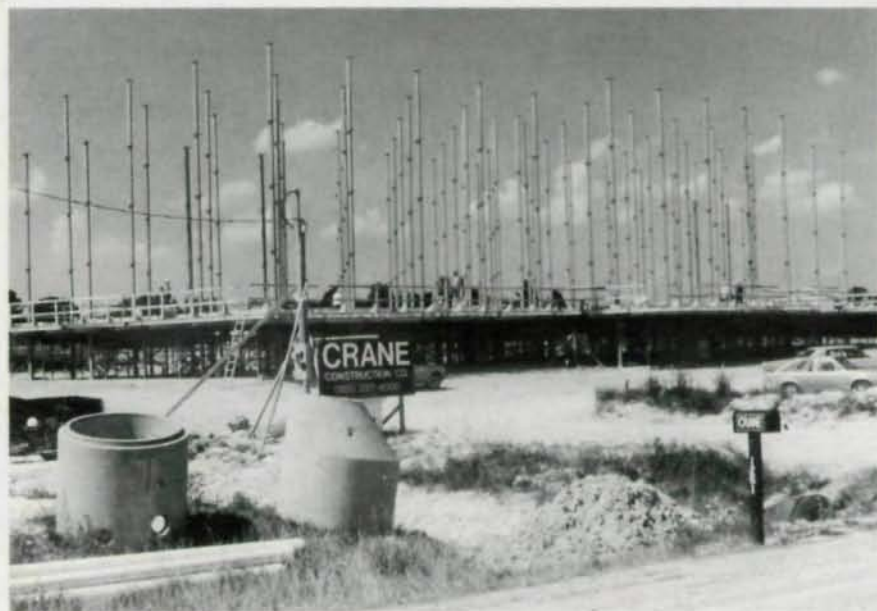
With an innovative construction technique, five-story steel tube columns with steel plates spaced every 8½' are bolted to a concrete strip foundation (above and top left). Form work is then put in place and the first floor is poured (left).
