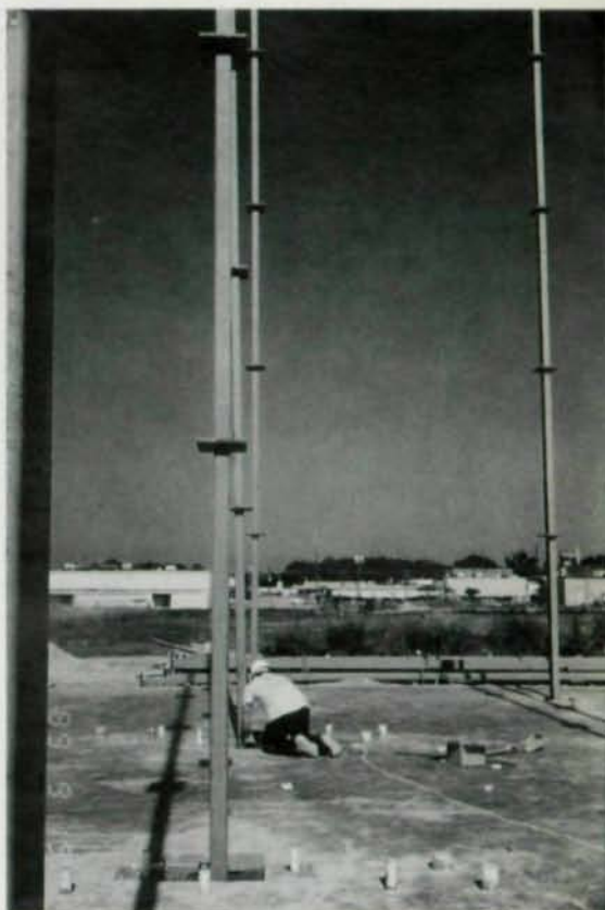
With an innovative construction technique, five-story steel tube columns with steel plates spaced every 8½' are bolted to a concrete strip foundation (above and top left). Form work is then put in place and the first floor is poured (left).
