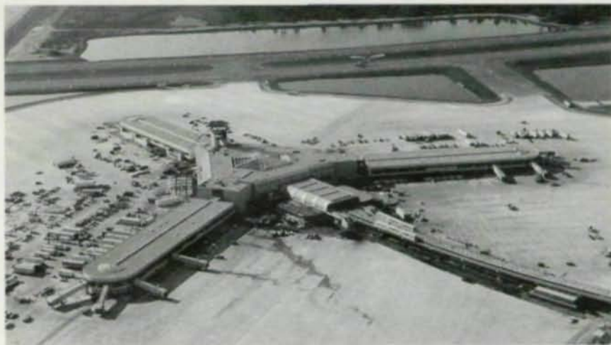
Delta Airlines Orlando Flight Center features a modern, sleek design and includes three 410'-long concourses surrounding a central hub. Top photo by Steven Brooke
