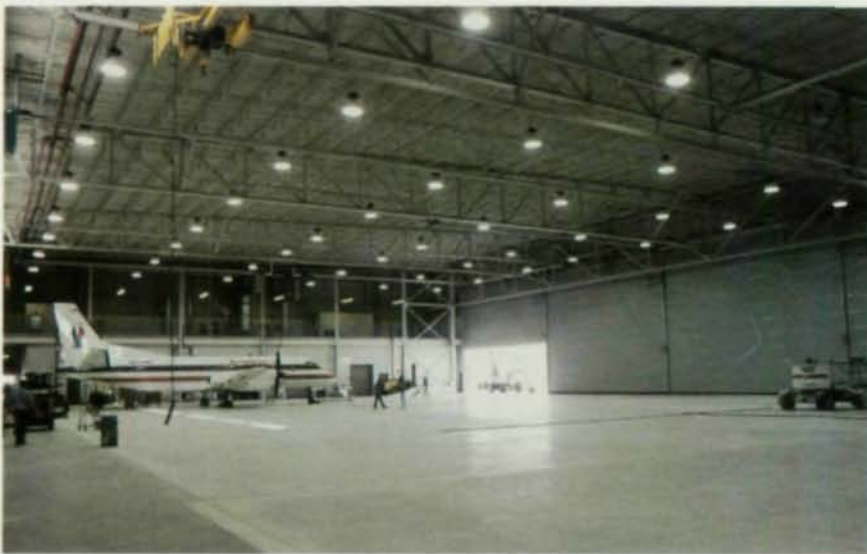
The hangar area for the new FFV Aerotech maintenance facility is 226'-wide by 150'-deep and provides space for three airplanes simultaneously.
