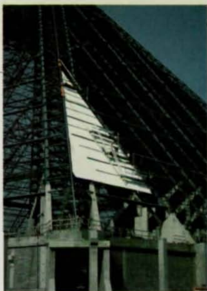
The four corners of the 290'-tall pyramid are framed with box trusses 14' wide and 18' deep. Each box truss is on a massive concrete wall buttress 24" thick and two-stories high.
