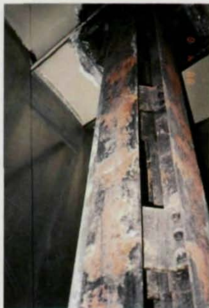
Many of the existing steel columns were strengthened with reinforcing plates on the flanges of the columns.
