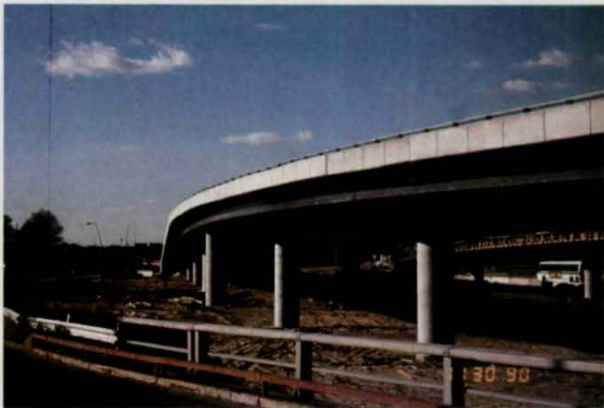
The new elevated roadway at John F. Kennedy International Airport in New York City was designed to easily handle the more than 5,000 vehicles arriving at the airport every hour.
