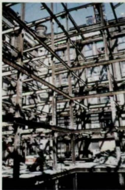
The entire structure above the second floor was renovated.
