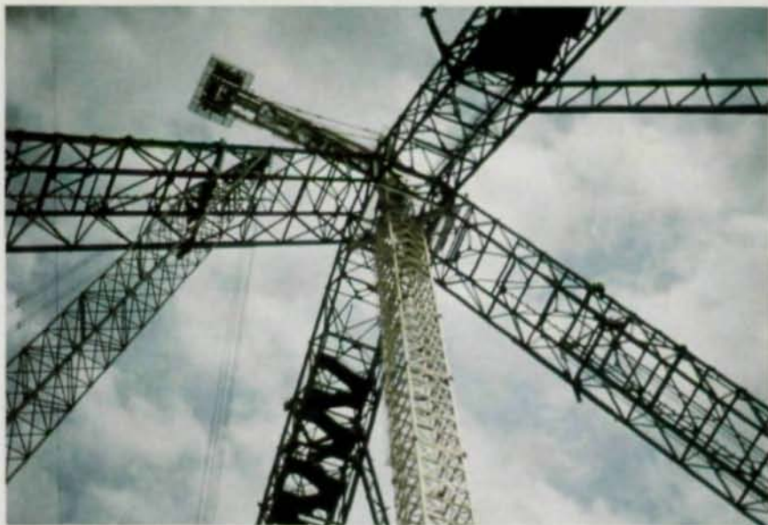
Metal stairs inside two of the four box trusses provide ground level access to the observation level. These structural steel stairs were fabricated and constructed prior to erection.
