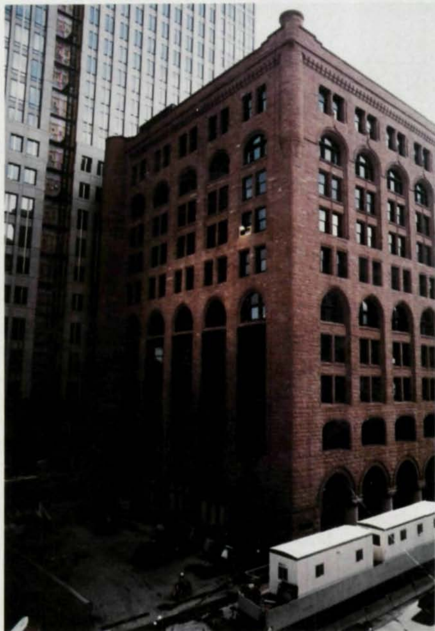
The interior of this 1888 building was completely rebuilt to create modern office space. Photography by Mort Tucker Photography.
