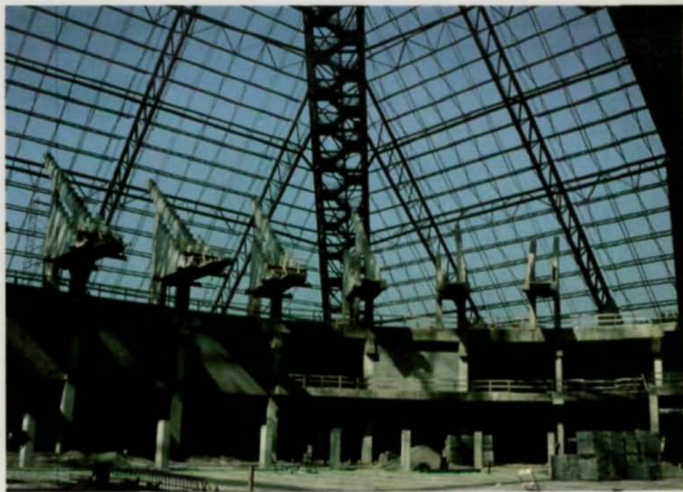
The four corners of the 290'-tall pyramid are framed with box trusses 14' wide and 18' deep. Each box truss is on a massive concrete wall buttress 24" thick and two-stories high.
