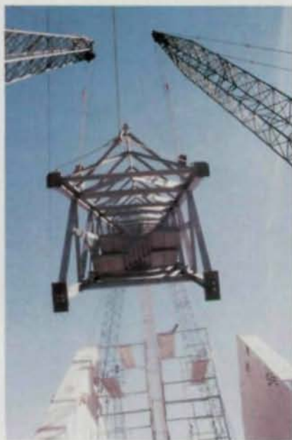
Metal stairs inside two of the four box trusses provide ground level access to the observation level. These structural steel stairs were fabricated and constructed prior to erection.
