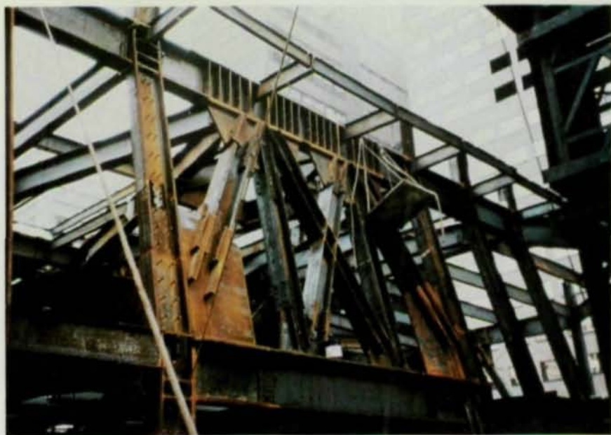
A construction photo of the sixth floor of the Mellon Bank Center in Philadelphia (above) reveals the sloping columns and trusses necessary to create column-free space. Shown at left are the upper floors of the 55-story building under construction.
