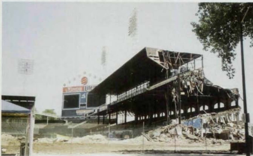
The steel from old Comiskey Park is being recycled into new wide flange sections.
