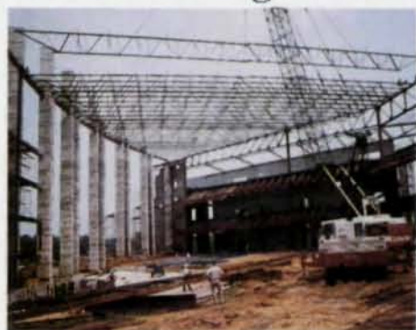
Our super long span joists easily bolt together on the job site.
