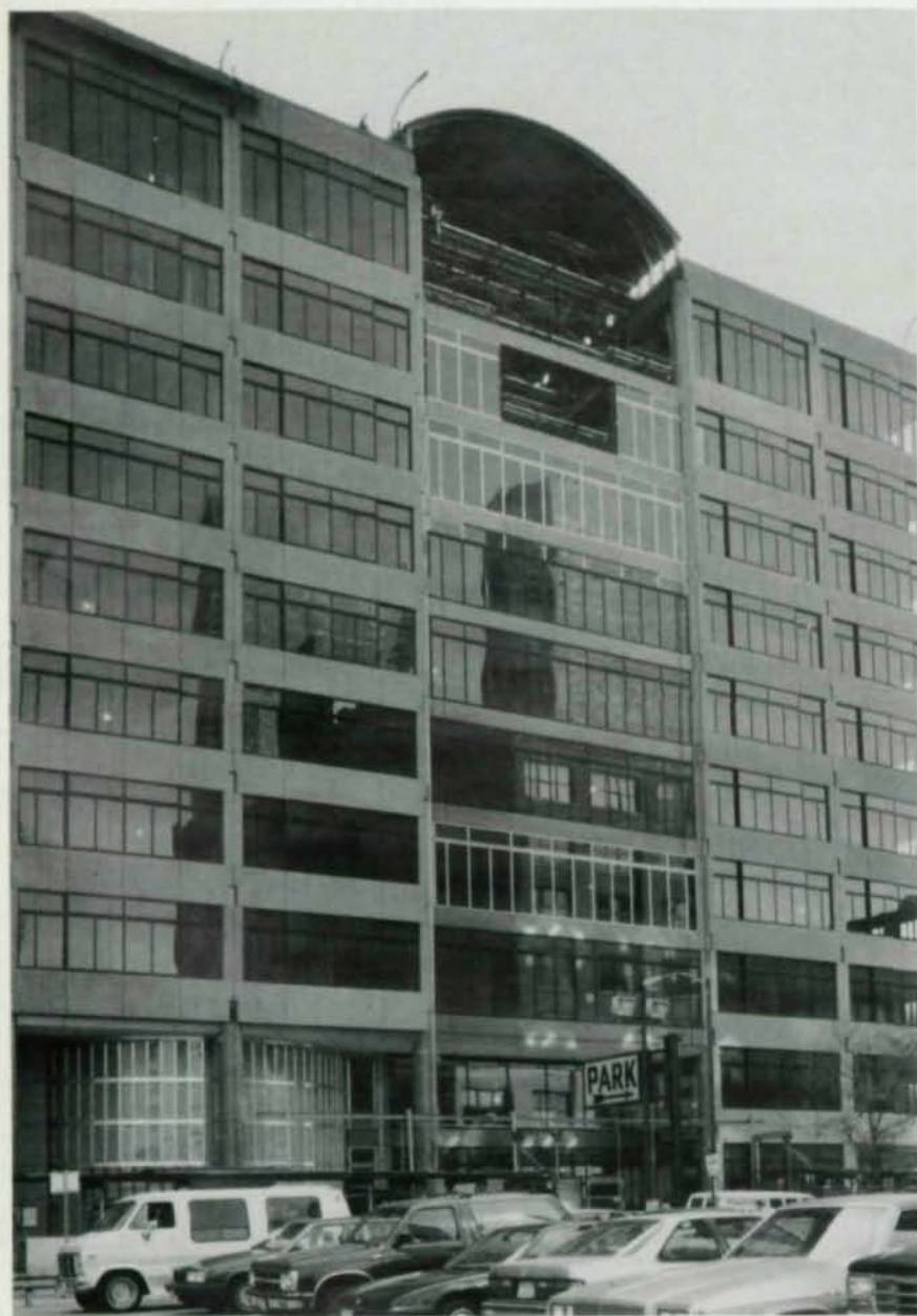
The 10-story building will contain classroom space on the lower three floors, leasable office space on the next two floors, and a library on the upper five floors.
