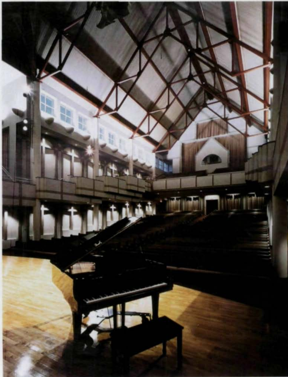
The chapel's exterior reflects the community's Dutch heritage, while the interior has a traditional church layout—but with the added twist of substituting exposed steel trusses for more traditional wood or stone architecture.
