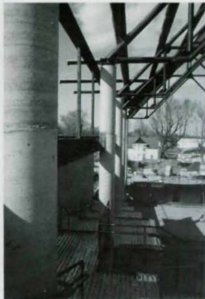
Connections were created by connecting the pipe to \frac{3}{8} " circular plates with fillet welds. Attached to the top of the trusses are 12" x 8" steel tubes, which support the wood roof deck.
