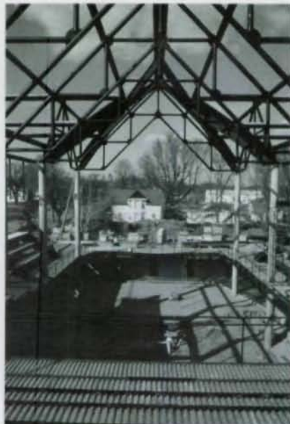
Connections were created by connecting the pipe to \frac{3}{8} " circular plates with fillet welds. Attached to the top of the trusses are 12" x 8" steel tubes, which support the wood roof deck.
