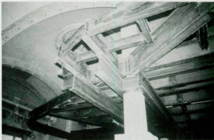
In the north wing, the mezzanine was cantilevered directly from existing columns (above and top). The mechanical trough (left) is supported on a box column formed with tubes in each corner connected with web members to form a truss assembly. Mechanical and electrical services run up the center of the column. Photos courtesy of Ryan-Biggs Associates.
