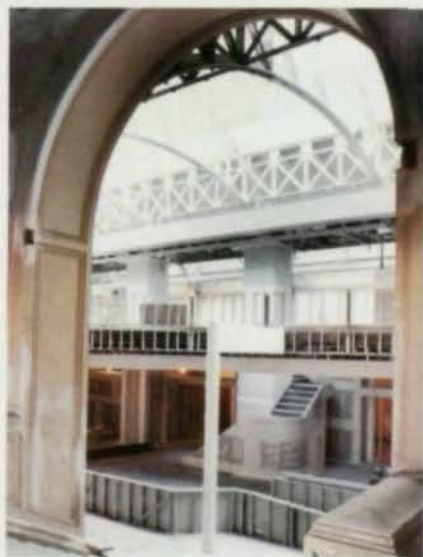
The new mezzanines are cantilevered off of tube columns that were attached to the structure's original steel columns. Extending from the steel tubes are short outriggers. Photo above by Jeff Goldberg/ESTO Photographics, Mamaroneck, NY; right photo courtesy of Eihorn Yaffee Prescott, P.C.
