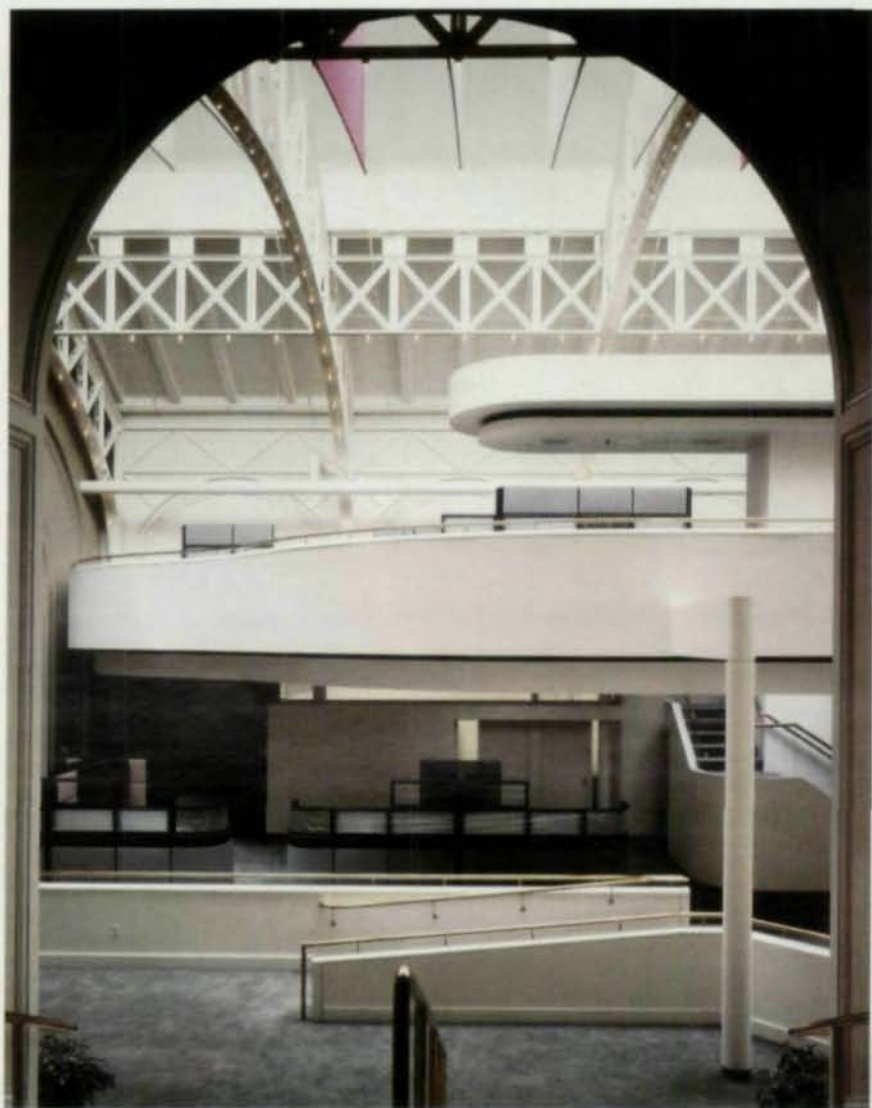
The new mezzanines are cantilevered off of tube columns that were attached to the structure's original steel columns. Extending from the steel tubes are short outriggers. Photo above by Jeff Goldberg/ESTO Photographics, Mamaroneck, NY; right photo courtesy of Eihorn Yaffee Prescott, P.C.
