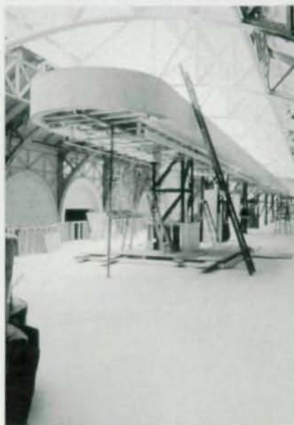
In the north wing, the mezzanine was cantilevered directly from existing columns (above and top). The mechanical trough (left) is supported on a box column formed with tubes in each corner connected with web members to form a truss assembly. Mechanical and electrical services run up the center of the column. Photos courtesy of Ryan-Biggs Associates.
