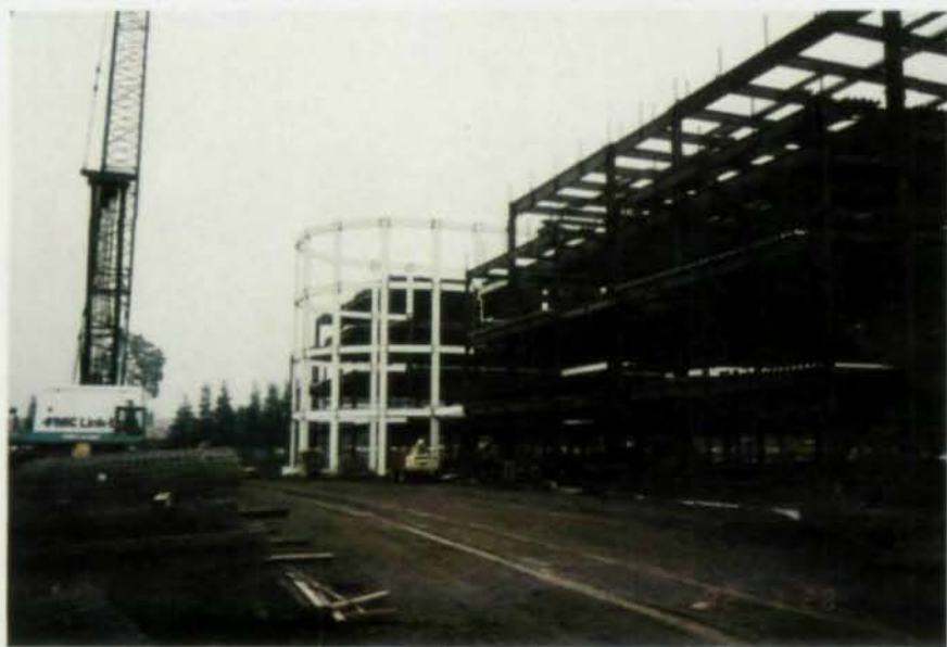
Each of the five four-story buildings of the Apple R&D Center consists of two wings with two Eccentrically Braced Frames in each wing and Special Moment Resisting Frames located at the building's perimeter.
