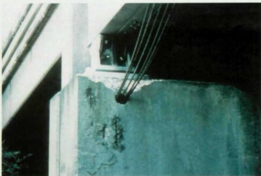
Figures 1 & 2: Cable restraining systems were added to older bridges to prevent girders from coming off of their supports during an earthquake.
