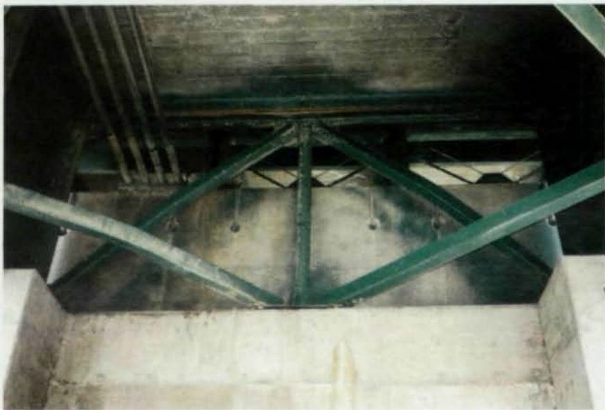
Figures 5 & 6: Figure 5 shows the north end of the main girder span of the Van Duzen River bridge after the April 25-26, 1992 tremors. Note that the restrainer cables on the left side of the girder is slack, while the cables on the right side are taut, indicating a movement to the left. Figure 6 shows a buckling of the lateral bracing system on the same bridge.
