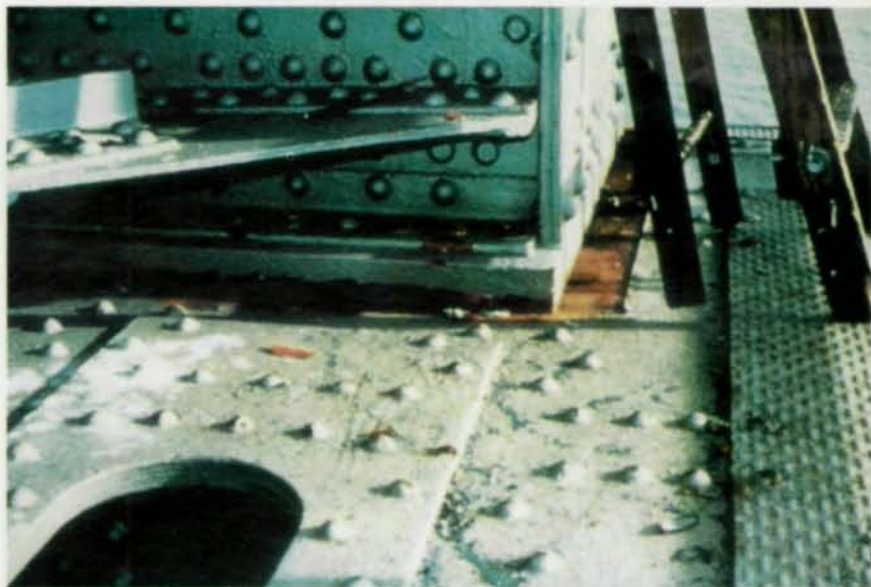
Figures 3, 3A, & 4: Figure 3 shows the damaged truss end post/lower chord bearing of the Bay Bridge after the Loma Prieta earthquake. Figure 3A shows a damaged backup bumper system on the same bridge. Figure 4 shows a typical seismic retrofit collar on an elevated viaduct.
