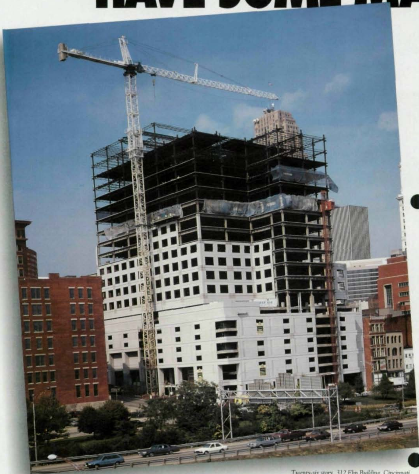
Twenty-six story, 312 Elm Building, Cincinnati.
