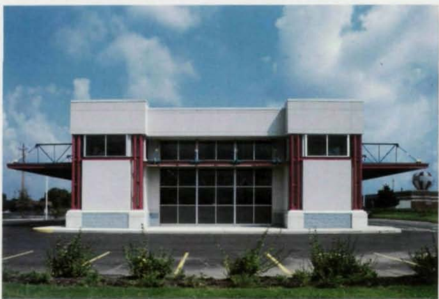
While the double-column (above and opposite) was initially designed for architectural reasons, it ultimately proved useful in simplifying the joist girder erection. Essentially, the girders sit on a plate saddle between the two columns. Photos by Jeffrey Jacobs/Nims Studios
