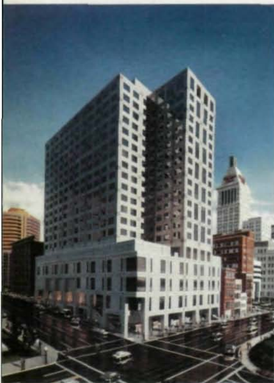
The framing system for 312 Elm in Cincinnati was selected both to minimize costs and maximize flexibility.
