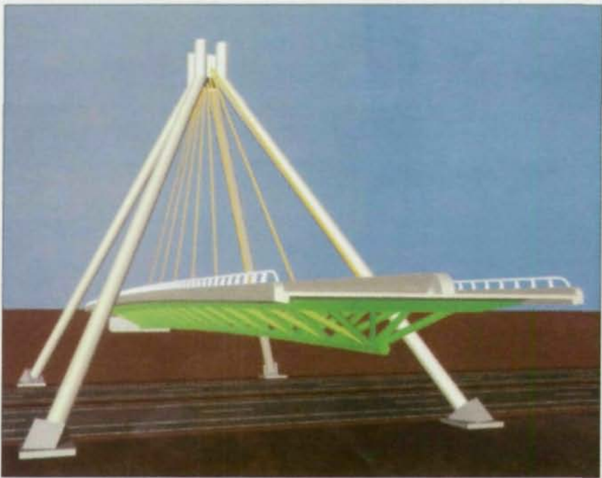
The top photo shows the completed Roize bridge, while the second photo is a CAD rendering of a potential future application (Figure 4a). Shown is a cable-stayed bridge where the cable-stays are anchored in the transverse center of the cross section. The stays are anchored at the apex of a four-legged pylon, creating a unique appearance.
