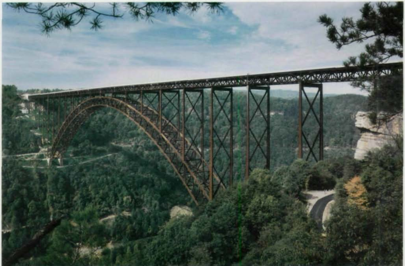
The New River Gorge Bridge in Fayette County, WV, is the world's longest steel arch span at 1,700'. It was constructed of weathering steel to minimize maintenance requirements and enhance its appearance. It was completed in 1977 at a cost of $35.2 million. Photo courtesy of Michael Baker Jr., Inc., a subsidiary of Michael Baker Corp.
