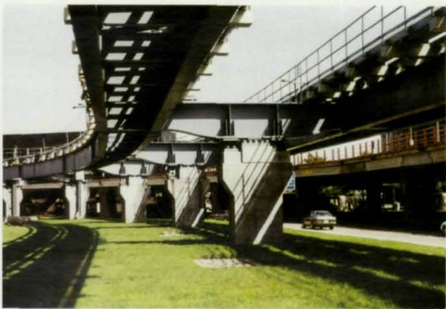
Above- and below-ground congestion necessitated wide-spaced guideways with narrow piers. The guideways are supported by wing-shaped crossheads that pierce the web of the inner guideway girders.
