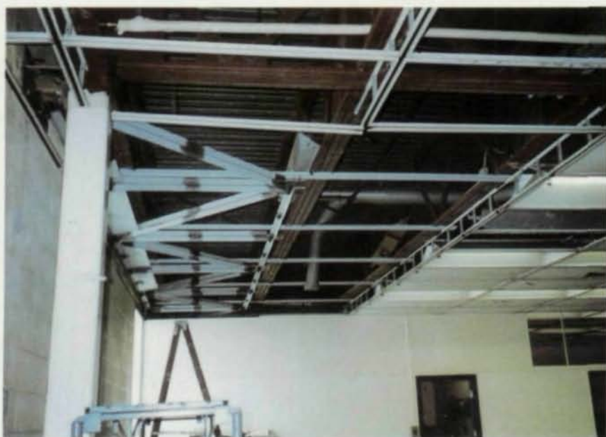
Figure 4: Completed Wind Truss
