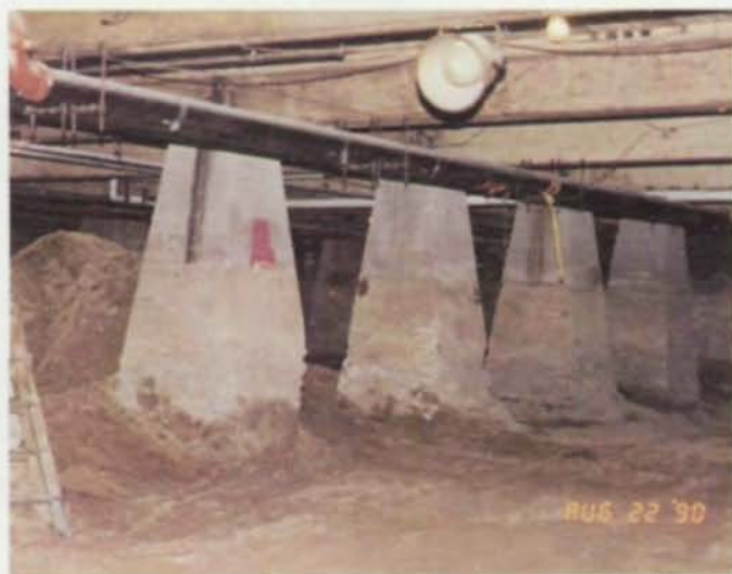
Shown at left is the crawl space below the existing first floor after excavation around the large concrete foundation piers. Shown below is the newly framed addition.
