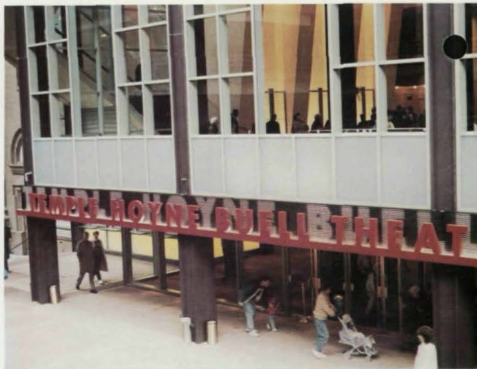
The theater's new lobby features a large glass wall overlooking a galleria connecting it to the Denver Arts Center.
