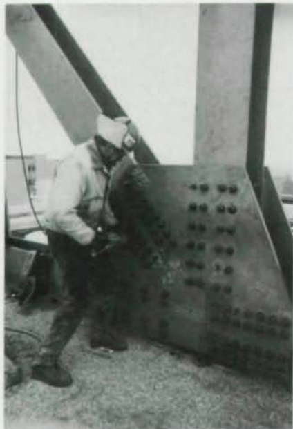
Due to its size and the lack of accessibility to its location, the large truss was installed in sections using bridge erection techniques (see photo at right).
