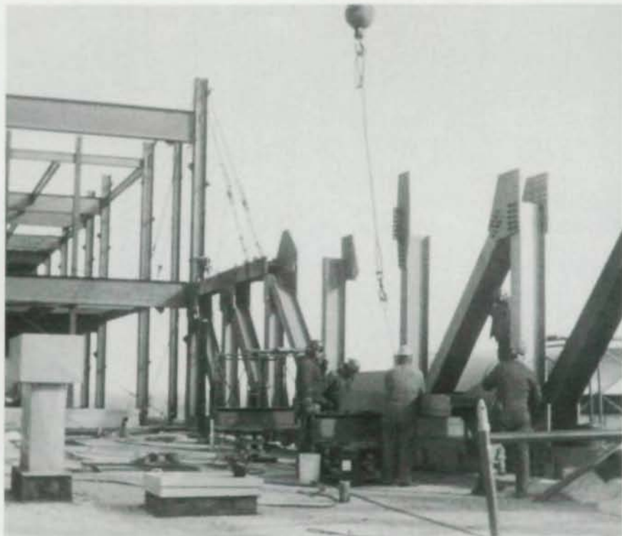
Due to its size and the lack of accessibility to its location, the large truss was installed in sections using bridge erection techniques (see photo at right).
