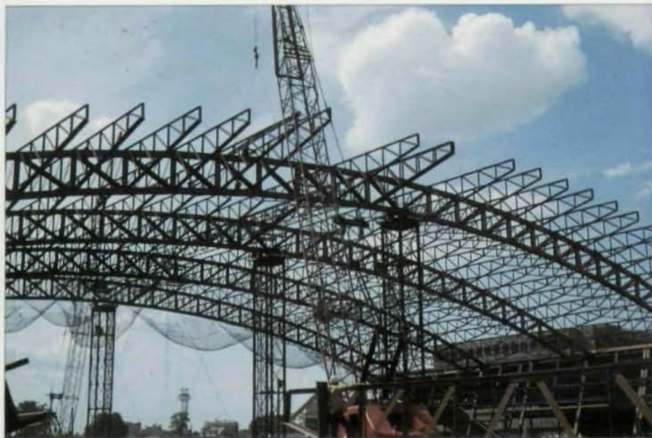
The Niagara Falls Convention Center featured eight steel arch-rib space trusses spanning 365' (111m) (shown under construction in the upper photo and completed in the lower photo). Zetlin developed quite a reputation for his work on long-span structures, starting with an Airplane Hangar at JFK International Airport in 1953 and continuing with his work on such notable structures as the Utica Auditorium and the Salt Lake County Civic Auditorium. In fact, it was the Utica Auditorium that first brought national attention to his fledgling design firm. Zetlin had a very creative mind, according to Max Abramovitz, FAIA, an architect who worked with him on several projects. "If you had a problem, he brought up creative answers to the problem, not the same old ordinary answers."
