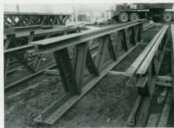
A composite joist system was used on the system because of its ability to handle the project's numerous large ducts while still maintaining a tight floor-to-floor height.
