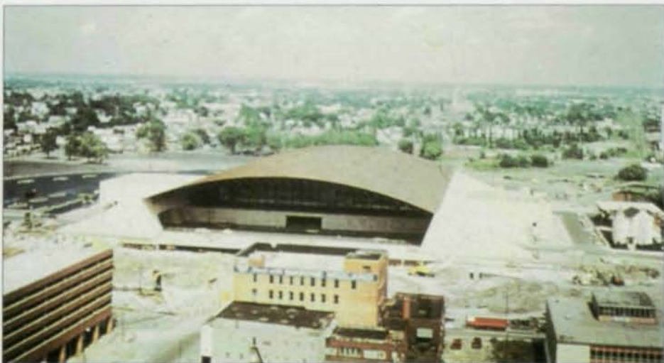
The Niagara Falls Convention Center featured eight steel arch-rib space trusses spanning 365' (111m) (shown under construction in the upper photo and completed in the lower photo). Zetlin developed quite a reputation for his work on long-span structures, starting with an Airplane Hangar at JFK International Airport in 1953 and continuing with his work on such notable structures as the Utica Auditorium and the Salt Lake County Civic Auditorium. In fact, it was the Utica Auditorium that first brought national attention to his fledgling design firm. Zetlin had a very creative mind, according to Max Abramovitz, FAIA, an architect who worked with him on several projects. "If you had a problem, he brought up creative answers to the problem, not the same old ordinary answers."
