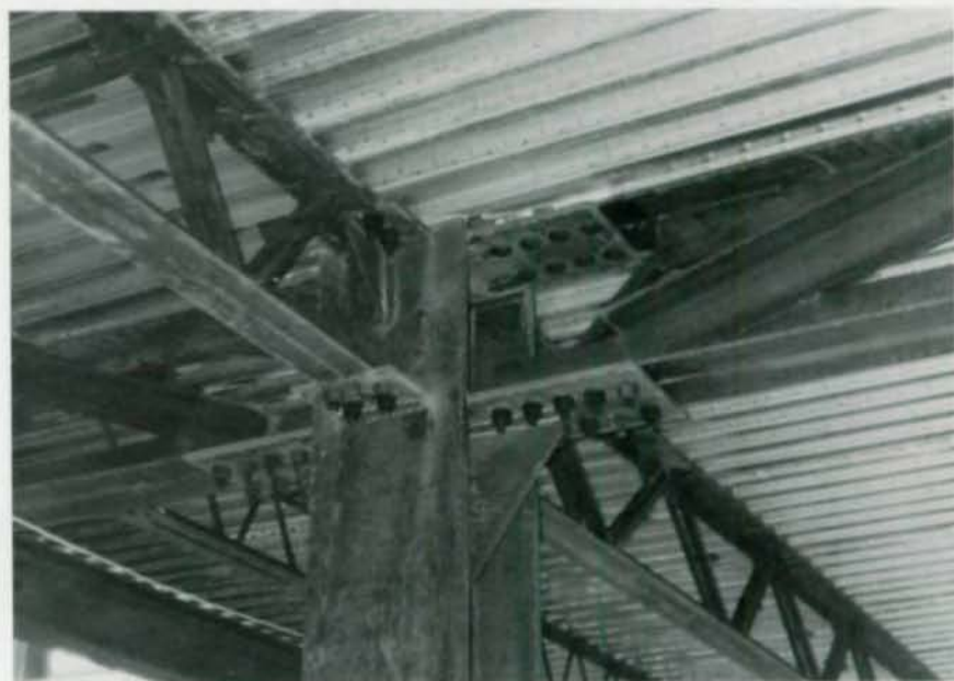
A composite joist system was used on the system because of its ability to handle the project's numerous large ducts while still maintaining a tight floor-to-floor height.
