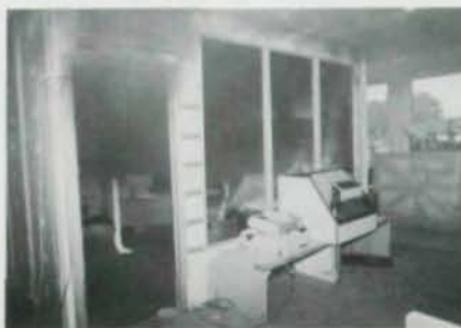
Water-filled drums were used to load the level 2 floor (top). A fire in the small office never spread beyond the room (bottom).
