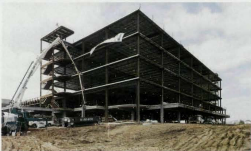
Switching from concrete to a steel frame saved Centrastate hospital approximately $1.3 million on its 135,000-sq.-ft. (12542m 2 ) addition.
