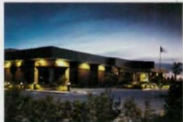
Tony Ingoglia Salami & Cheese Co., Sacramento, California, 25,000 sq. ft.; Architect/Engineer: Edward A. Bonelli & Associates; General Contractor: Holdener Construction Co.
