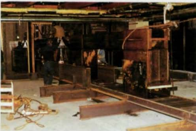
All of the steel was brought into the building during a weekend using a 250-ton crane. Members were hoisted up to the 15th floor and placed on a steel conveyor system, which extended 13' out of the window. Top photo by Boshke Photography.
