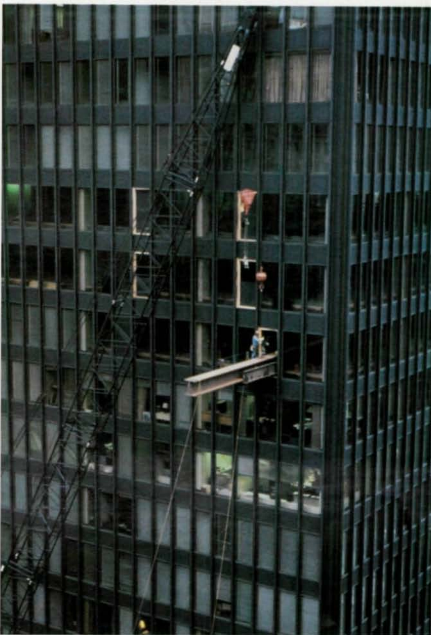
All of the steel was brought into the building during a weekend using a 250-ton crane. Members were hoisted up to the 15th floor and placed on a steel conveyor system, which extended 13' out of the window. Top photo by Boshke Photography.
