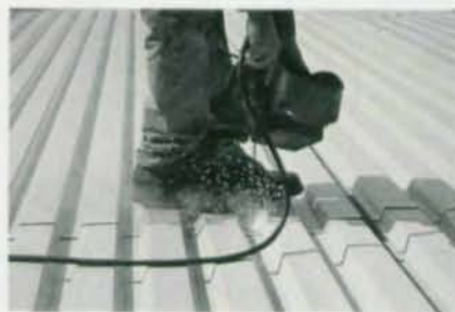
Welding of steel decks has a long track-record of success.
