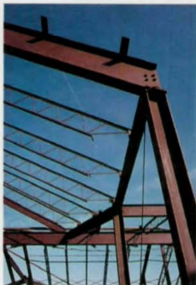
Sloped seat joists can be designed to fit almost any degree of pitch.
