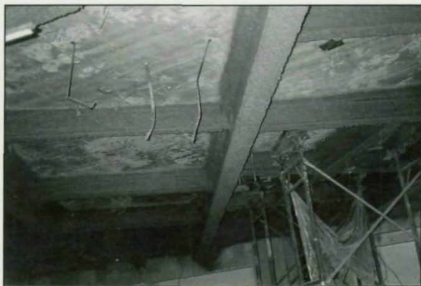
Shown above is the grid of new steel beams after fire proofing was applied.
