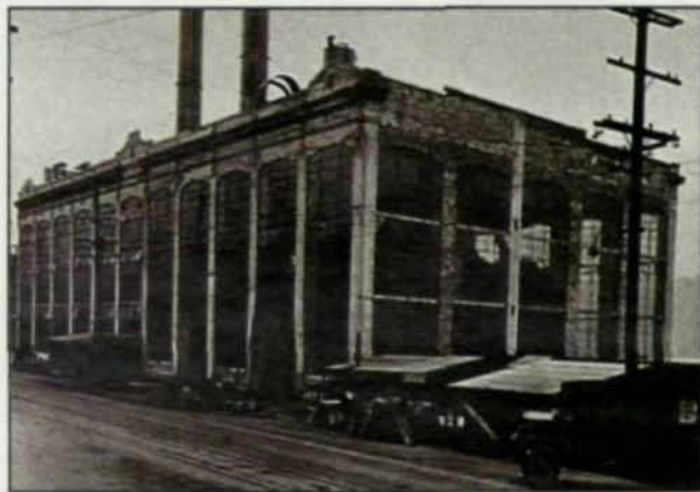
Three stages of evolution: the original steam plant under construction (top left); after completion in the 1920s (middle left); and as it looks today (opposite).
