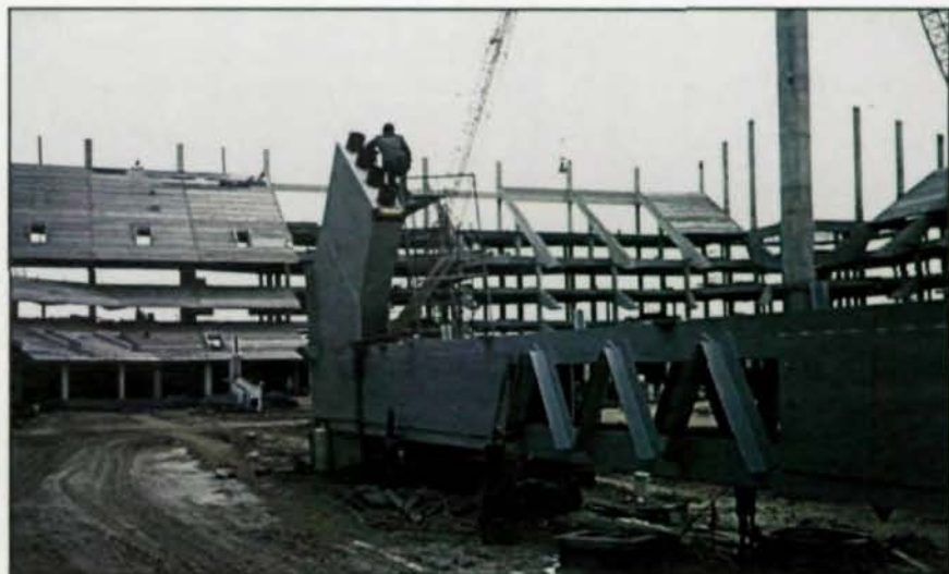
(Left) The outside tieback truss was held in place by the crane until cables were installed.
