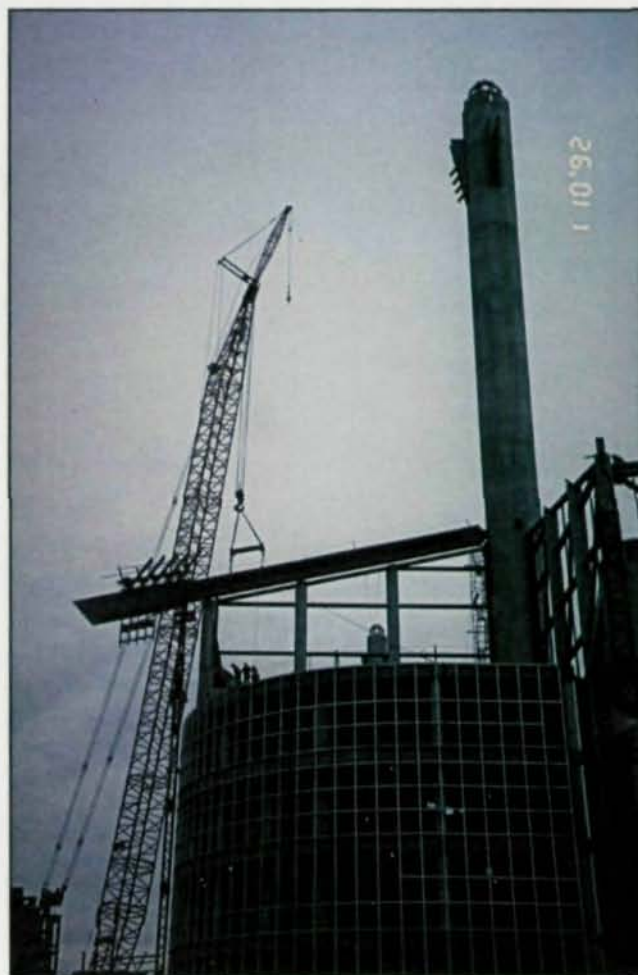
(Left) The outside tieback truss was held in place by the crane until cables were installed.
