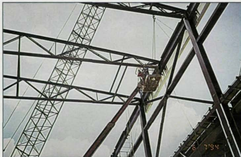
Spanning across the 200-ft. by 420-ft. practice space are large bow-string trusses. These joists, which are spaced 197-ft. on center, range in depth from 120-in. at the midspan to just 24-in. at bearing points.
