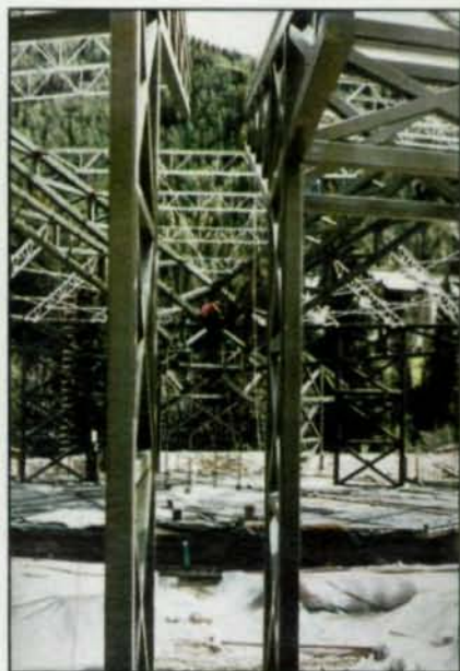
The Gerald Ford Amphitheatre in Vail, CO, features a roof with large cantilevers and utilizes free-standing roof and wall column sections that are designed to resist heavy wind and snow loads.
