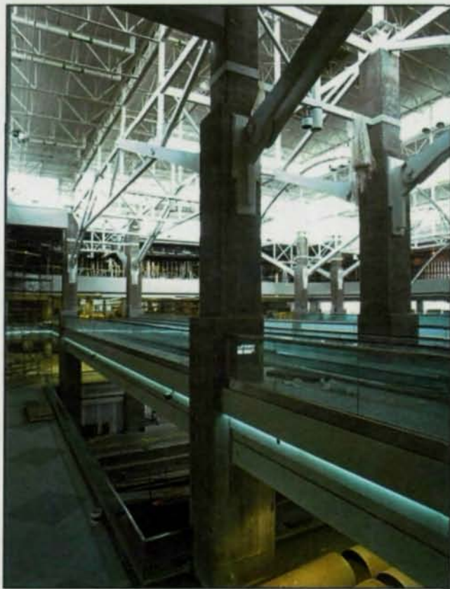
Pictured above is a view of the exposed roof in Concourse "C" at the new Denver International Airport. Shown at right is a view of the typical roof framing in Concourse "B", including the aptly named "Hero" trusses.
