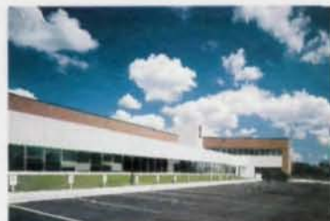
Station KMSP-TV, Eden Prairie, Minnesota, 36,000 sq. ft.; Architect: Korsunsky Krank Erickson; Consulting Engineer: Nelson-Rudie & Associates; General Contractor: Kraus-Anderson Construction Co.; Steel Fabricator: Central Minnesota Fabricating; Steel Erector: Amerect, Inc.
