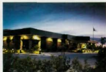
Tony Ingolia Salami & Cheese Co., Sacramento, California, 25,000 sq. ft.; Architect/Engineer: Edward A. Bonelli & Associates; General Contractor: Holdener Construction Co.
