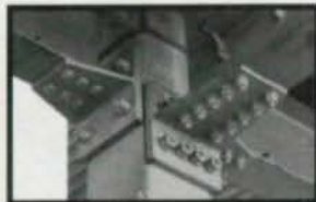
Detail of actual box column-to-beam connection using Huck ULTRA-TWIST fasteners.
