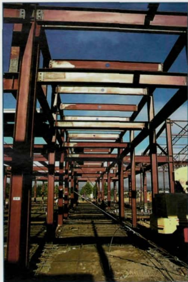
A steel frame was selected for the Alameda County Office of Emergency Services / Emergency Operations Center because of space planning flexibility, opportunities to feature exposed framing in the architecture, speed of erection and proven earthquake performance
