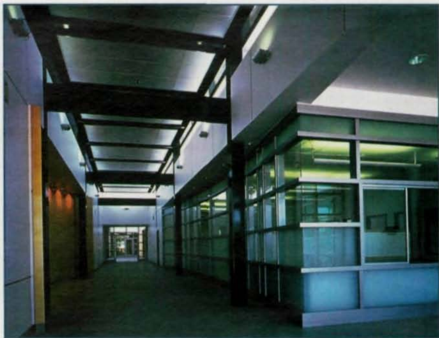
A steel frame was selected for the Alameda County Office of Emergency Services / Emergency Operations Center because of space planning flexibility, opportunities to feature exposed framing in the architecture, speed of erection and proven earthquake performance
