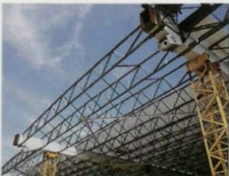
90' Vulcraft steel joists.
